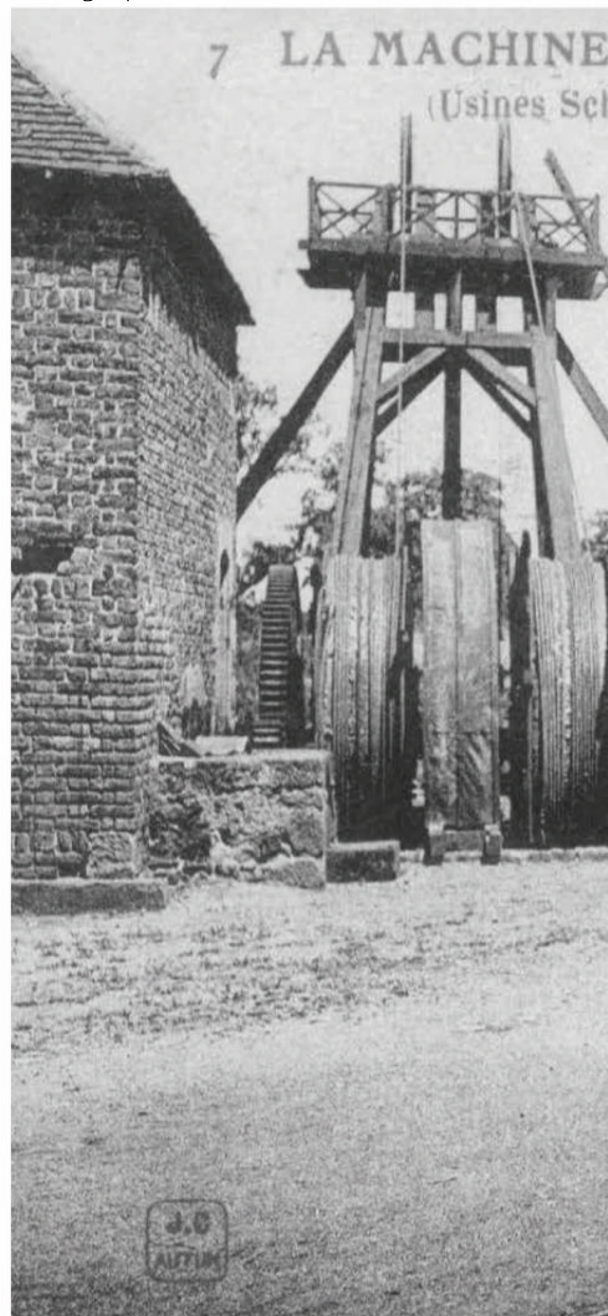
Shunting skips at La Machine.
