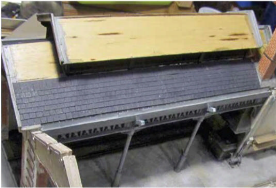
After having glued the bargeboards covered by zinc flashing, complete rows of slates are put in place.
