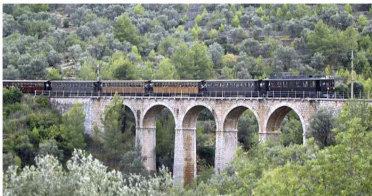
Viaduct/Cinq near Soller, 11th September 2001.
