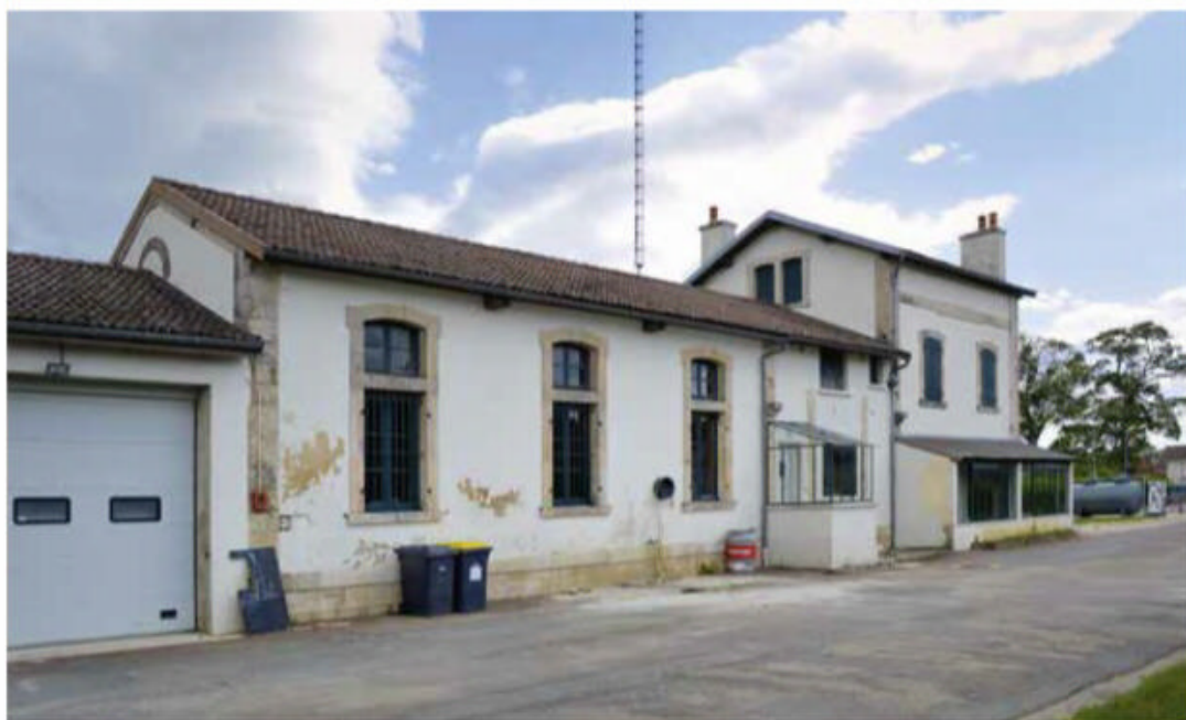
The long building at Baigneux-les-Juifs seen from the track side as it is nowadays, June 2019.
