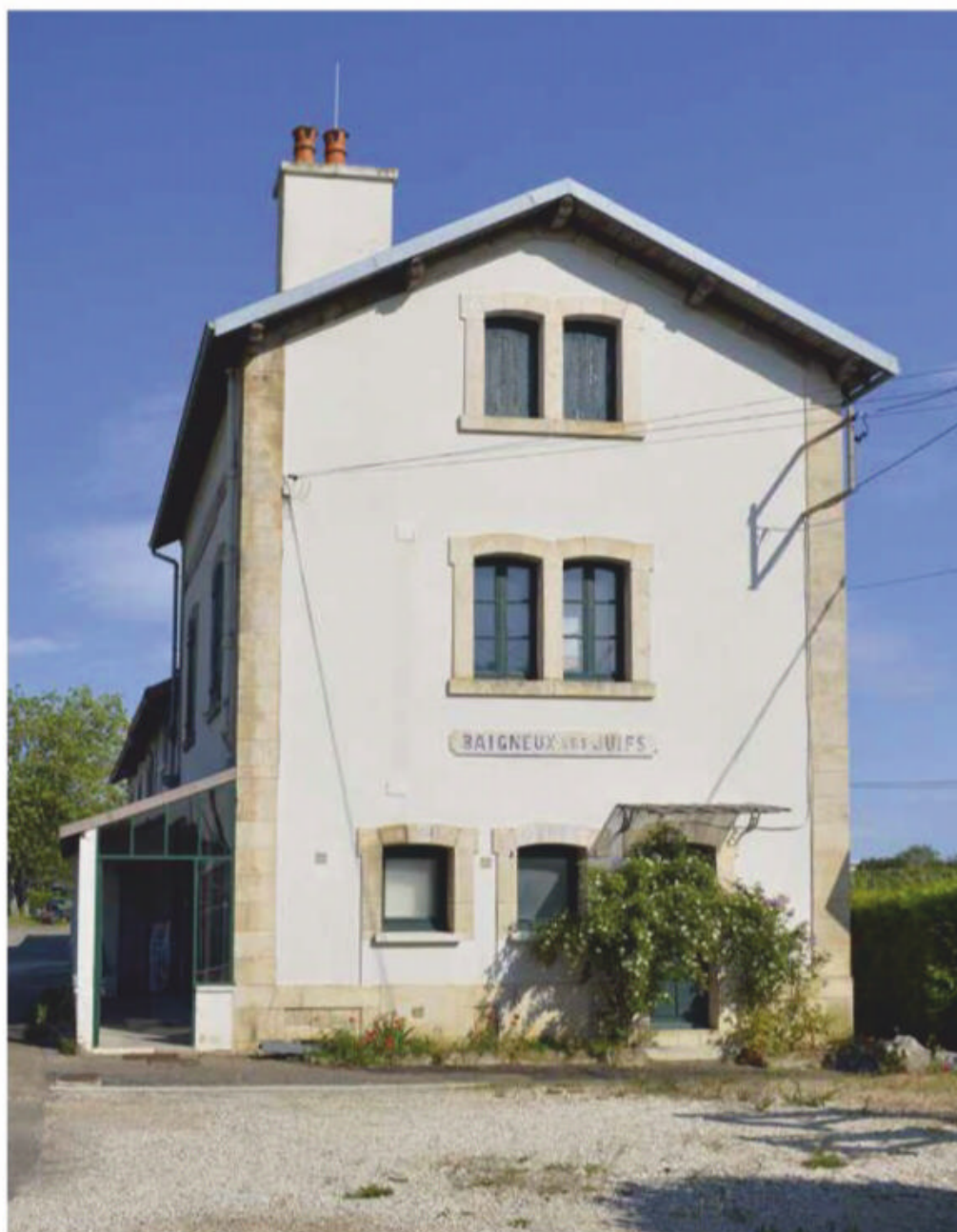
The gable of the passenger station building, June 2019.
