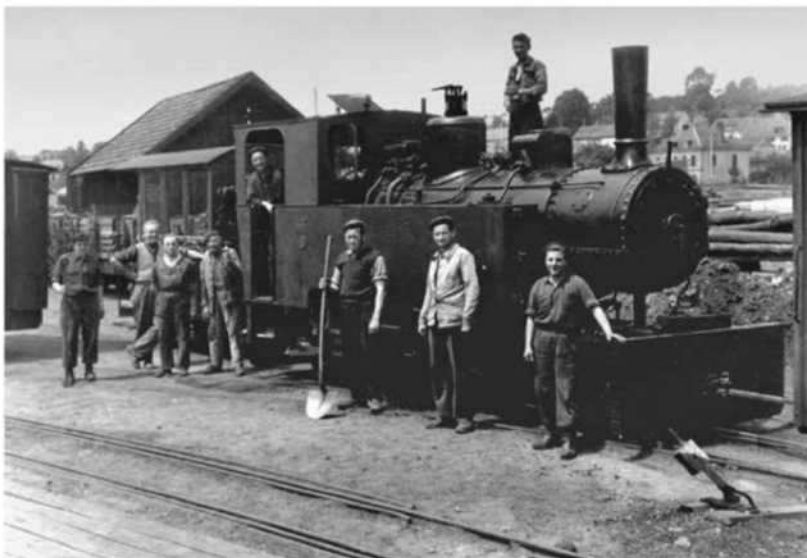
On the site of the Abreschviller sawmills, a driving crew takes a break in La Forge station.
