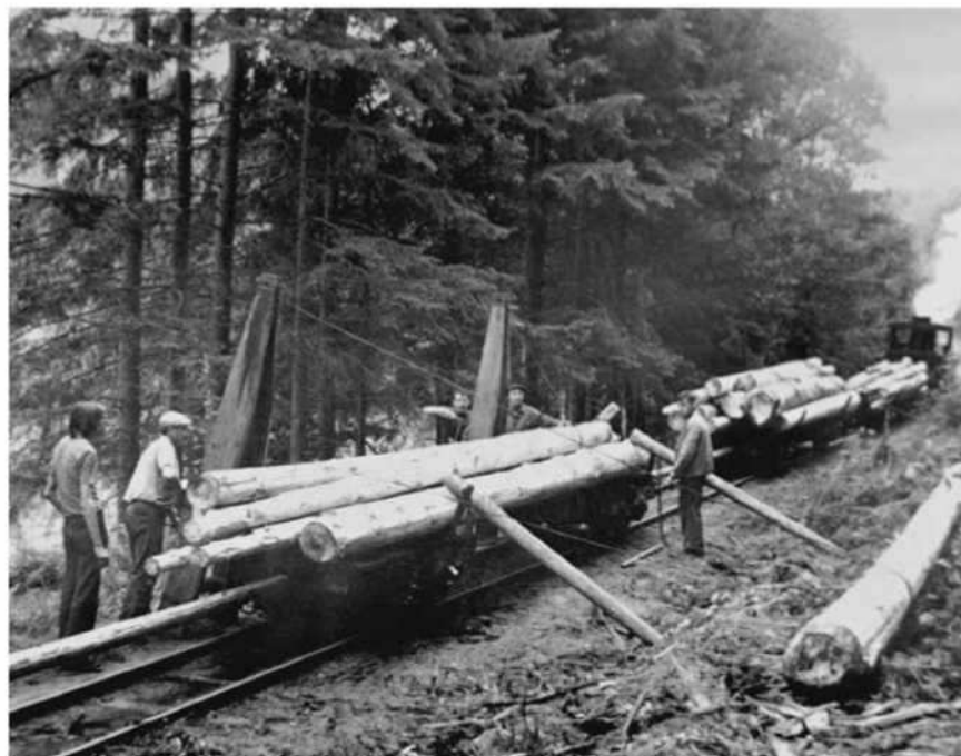
Loading a log with jacks at Saint-Luc.
