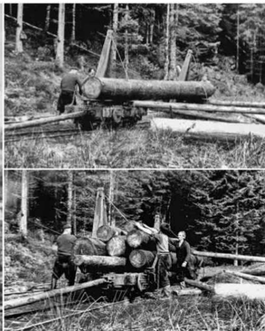
The loggers complete the loading of a pair of bolster trucks.
