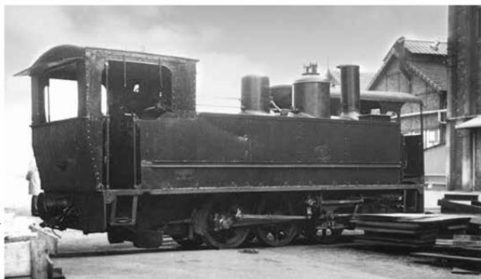
Pinguely 0-6-0 T locomotive N° 101 with reinforced water tanks, seen on the turntable at the forges in 1953. This engine was transferred to the Chemin de fer de la Baie de Somme in 1975 .
