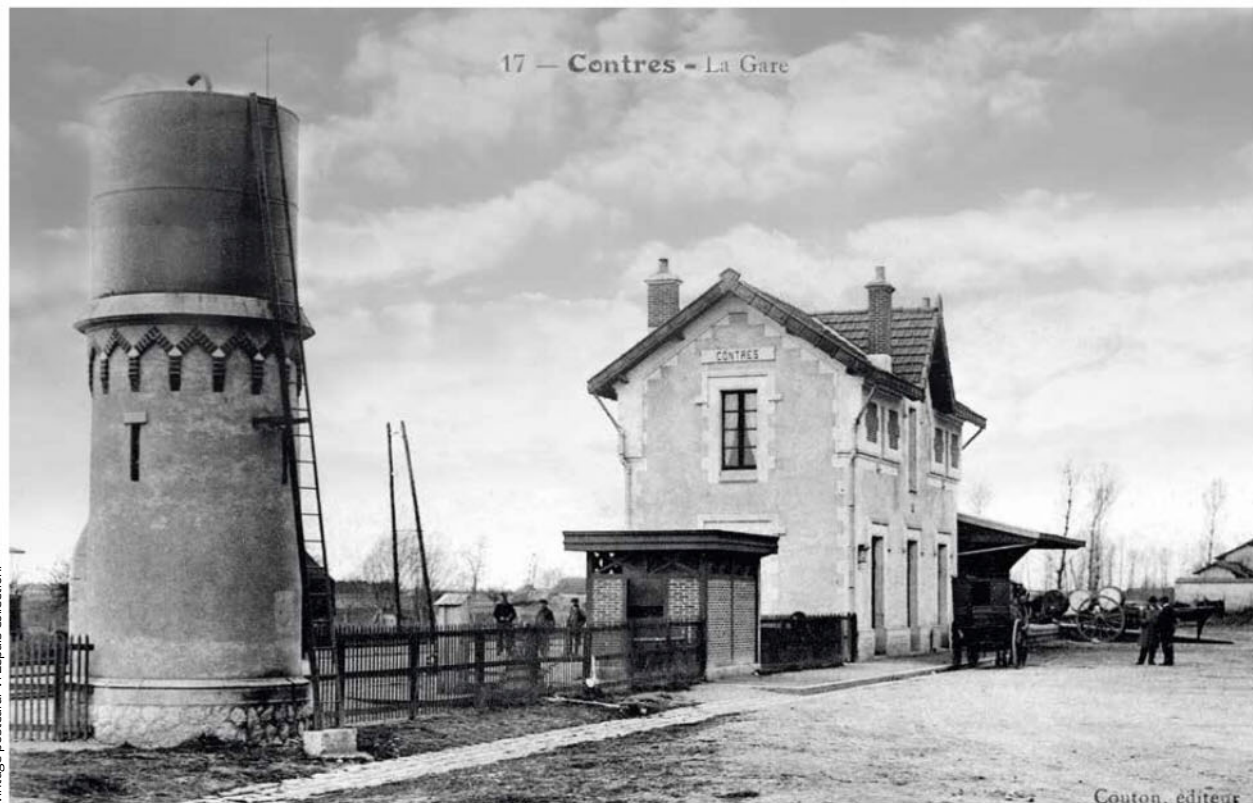
Contres station, admire the contouring that also graces the water tower.
