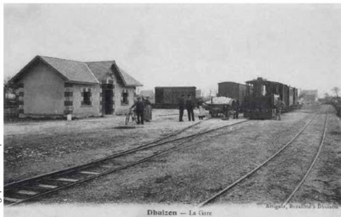
Dhuizon station, seen from the other end.
