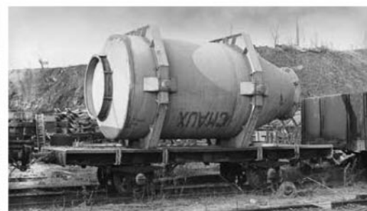
Flat wagon adapted for carrying lime, seen at the forges on 28 February 1968.
