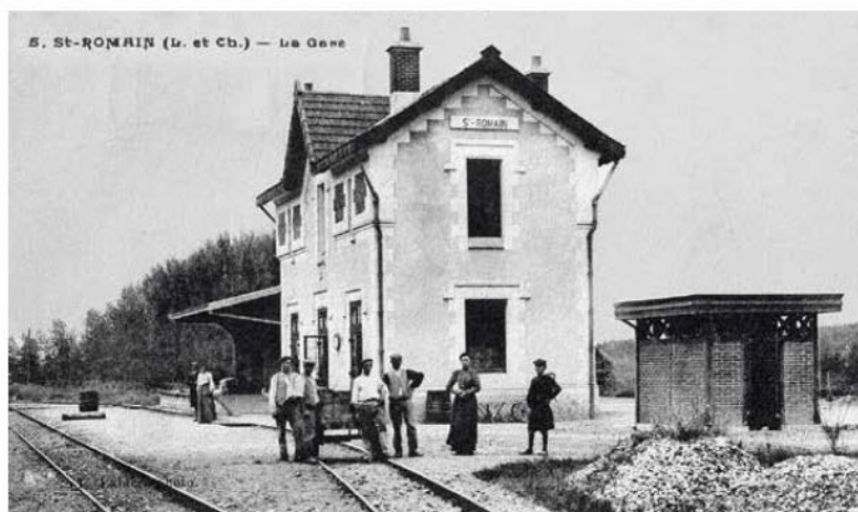
Saint-Romain station is built on the same pattern, seen here from the tracks.
