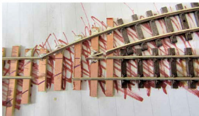
Soldering work begins.
