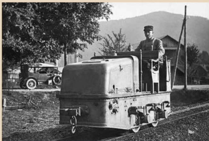
Wesserling, 8 August 1916, a petrol-driven motor-trolley on 60cm gauge track, used by the Engineer Corps.
