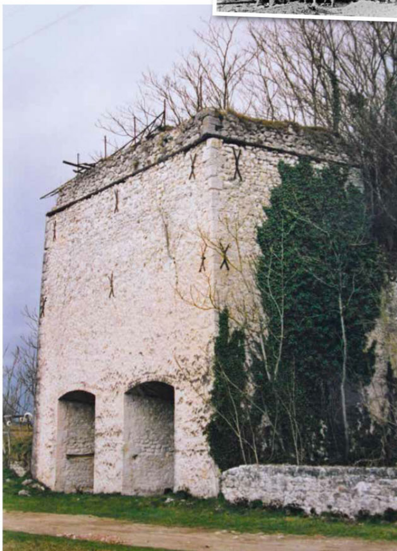
This overview shows the location of the kiln, which backs on to a hill. The top of the kiln featured railings to protect the workers. 28 February 1998.
