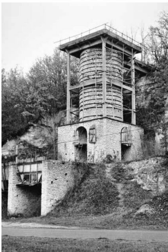
Another type of structure, but serving the same purpose, the Rochats lime kiln at Mauvières in the Indre. The lime is dumped out of the kiln into the loading chutes installed at the foot of the building. 10 February 1990.
