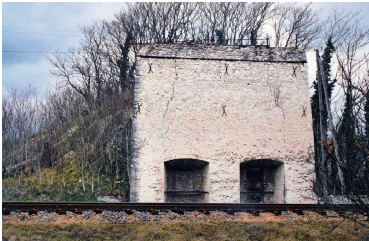
The South side of the kiln with the Blanc-Argent line in the foreground. The kiln has the appearance of a large block of masonry. 28 February 1998.
