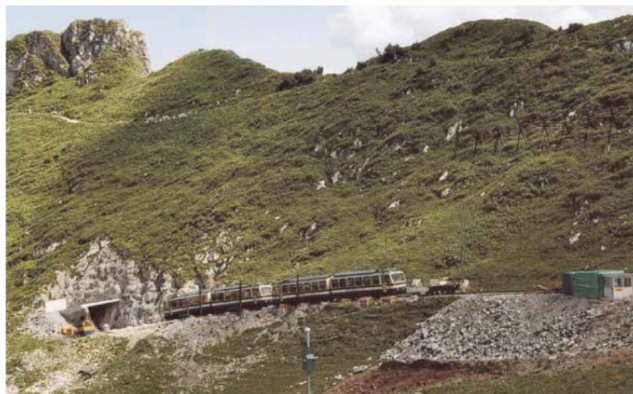
The motor units, operating in MU mode, have just emerged from the Naye gallery. 7 July 2010.
