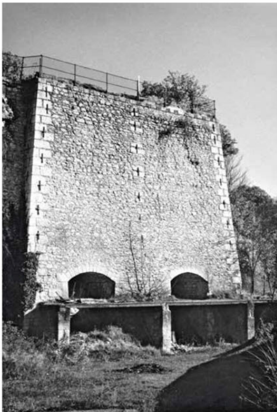
Terriers de Neuville lime kiln at Chasseneuil (Indre). The emptying platform is clearly visible. 11 November 1989.
