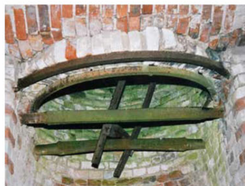
Under the segmental arched openings, the stokeholes are visible. The two cart axles, embedded in the masonry, used to support the grate. A length of narrow gauge Popineau track, dumped into the kiln, has been caught up by one of the cart axles. 28 February 1998.
