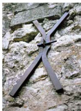
To withstand the high temperatures that would otherwise split the masonry, the kiln is reinforced by metal stays, whose anchors on the front of the structure are clearly visible. 28 February 1998.
