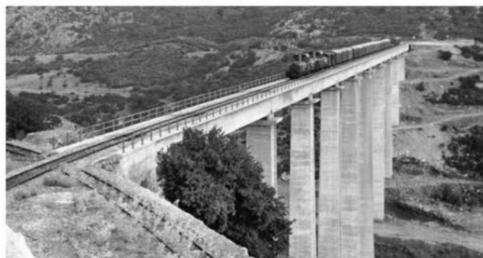
The rebuilt viaduct at Achaldokambos. 25 July 1975.
