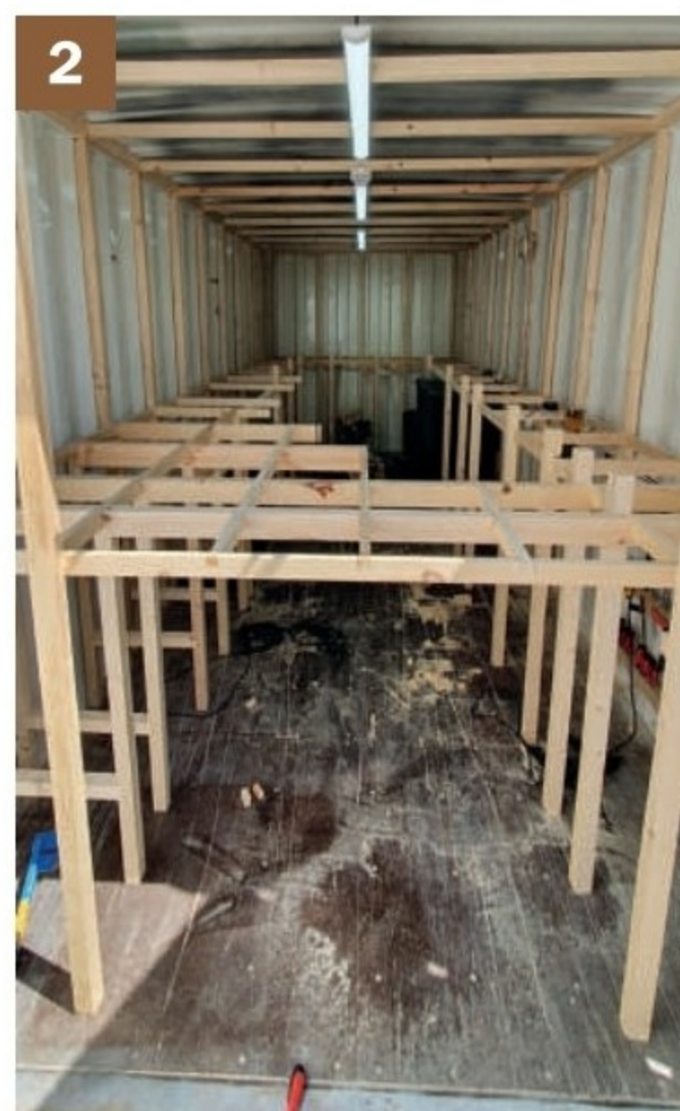
2 A substantial timber framework was constructed.
