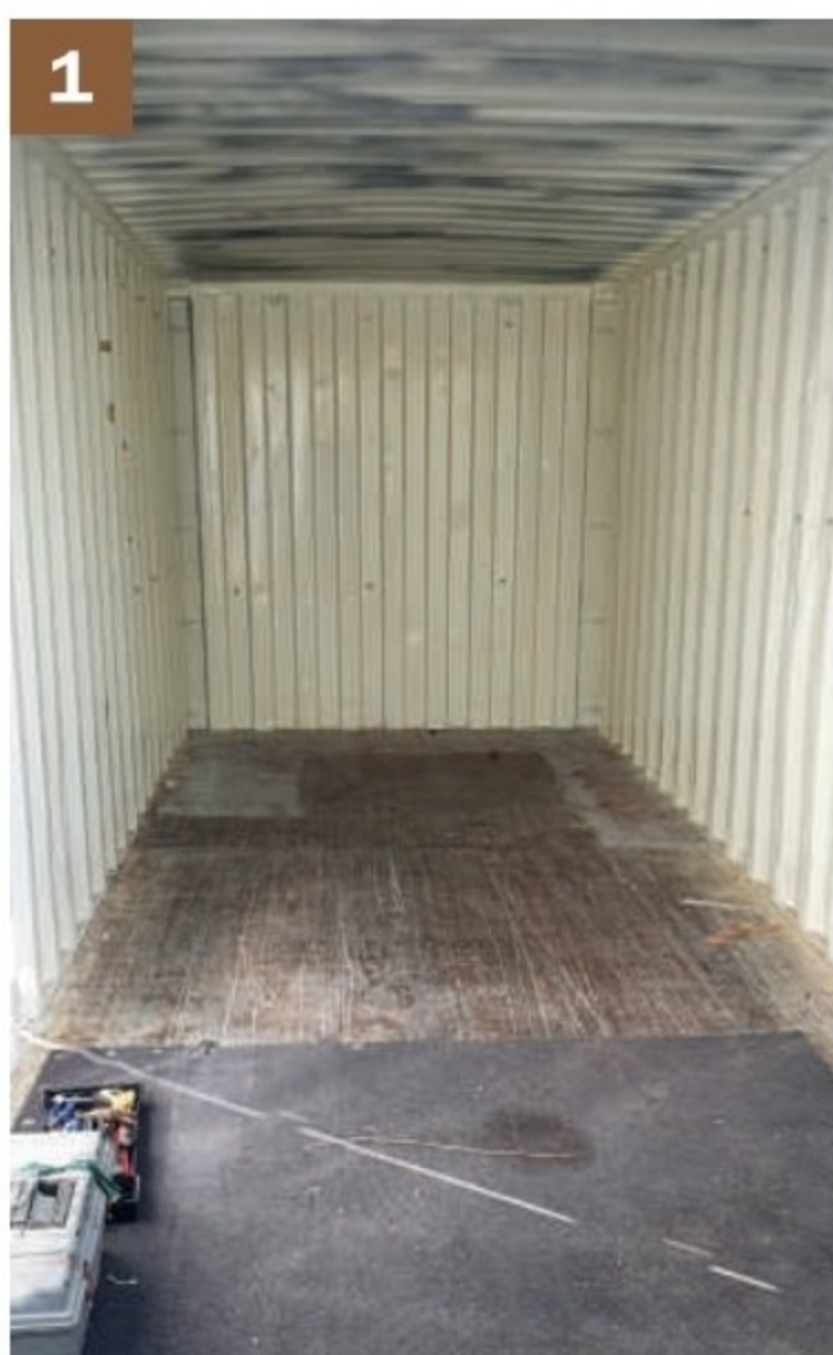
1 The interior of the shipping container prior to work commencing.
