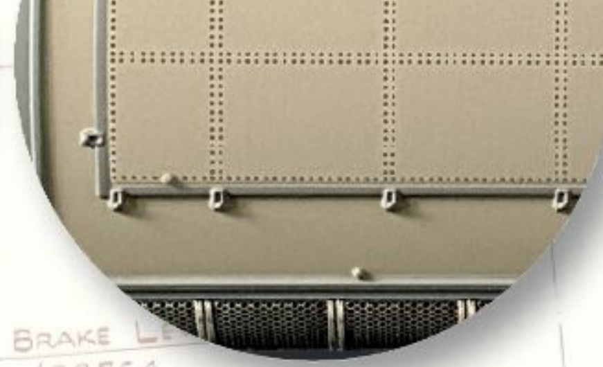
Rivetted roof panels
