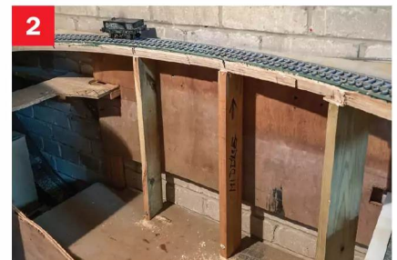
2 ▲ Timber uprights were installed to provide the arch supports.
