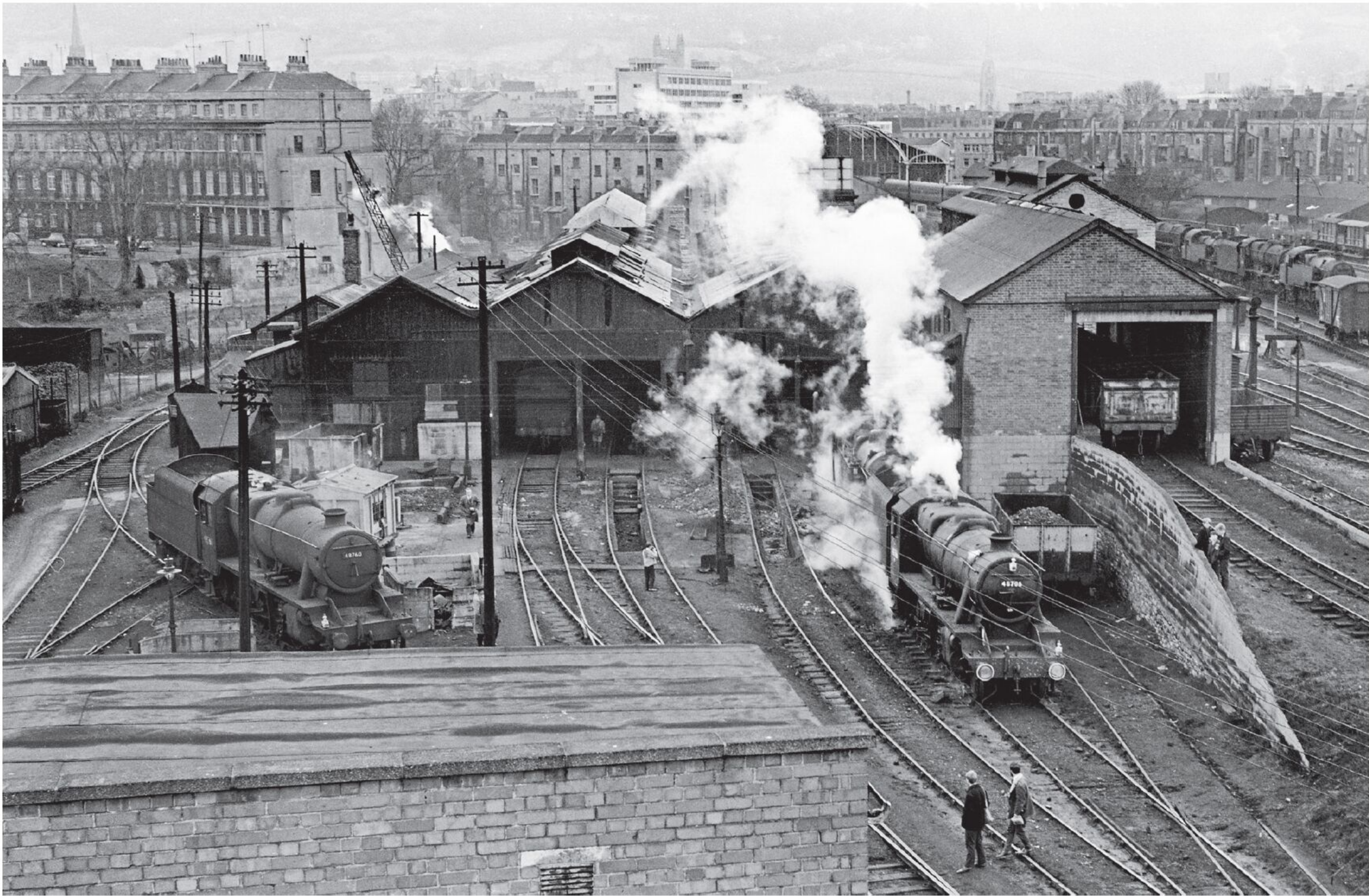
◀ An overall view of the S&D shed and yard at Bath Green Park on 5 March 1966 (the last day of public services on the S&D route). The two-road Midland shed can be seen above the brick-built coaling stage, to the left of which the overall roof of the station is visible. The two Stanier 8Fs are Nos.48760 (left) and 48706 (right). Photo: Rail Photoprints
