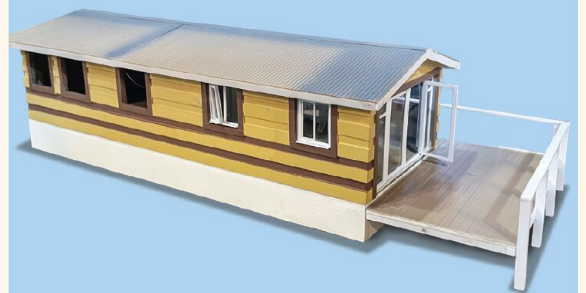
A brick base was added around the lower part of the caravan.
