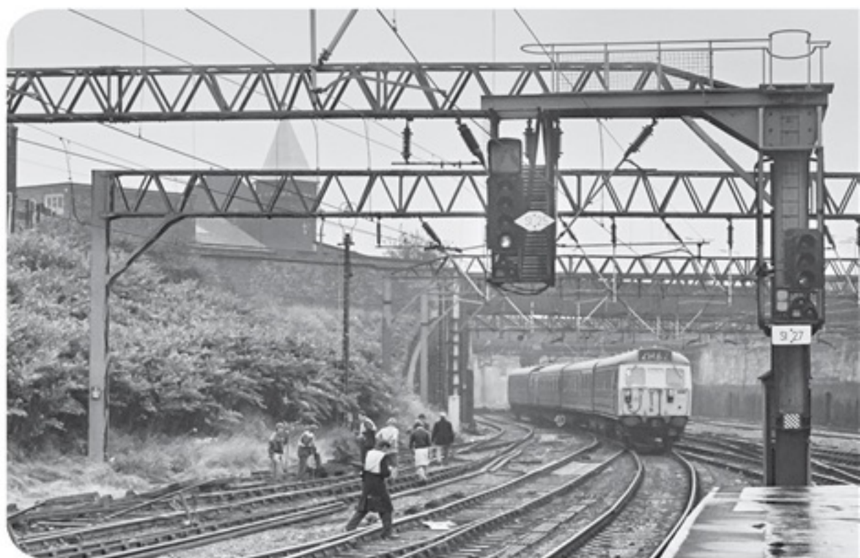
Above: Stockport in September 1976. The 25kV OHLE was of particularly sturdy construction on this early section of the WCML electrification project, and may be one possible reason why this section rarely features as a subject for modelling. Note also the attire of the rail workers, which is far removed from the high visibility protective wear demanded on today's railway.
