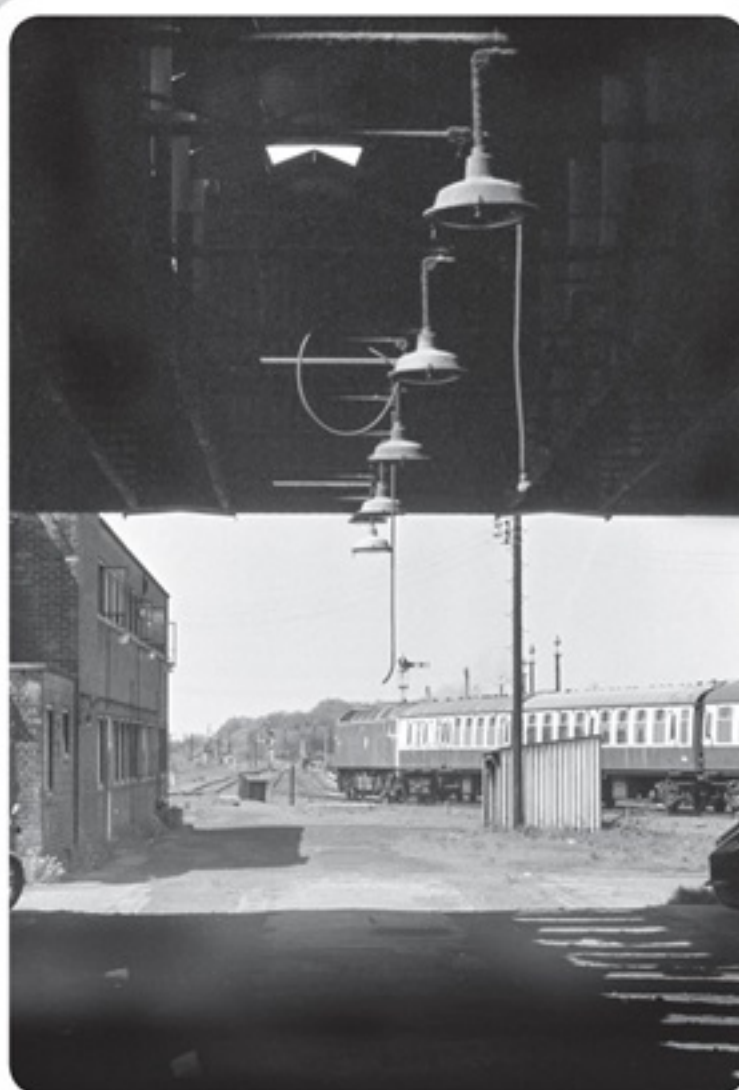
Above: Some steam age structures were not razed to the ground immediately after 1968. The ex GER/GNR shed at Lincoln (40A) was used for many years as a covered car park and is seen from within in May 1978 as an unidentified Class 47 heads westwards with a rake of Mk.1s. Both photos: Steve Flint
