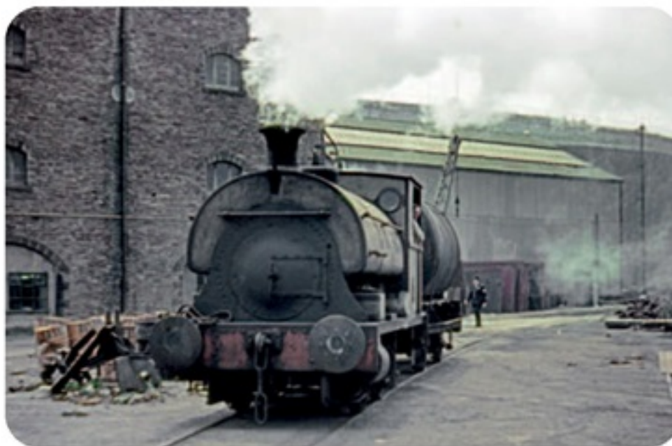
Above: Peckett 0-4-OST No.1530 shunting in Falmouth Docks in April 1970. The locomotive remained at work here until 1986. Photo: Rail Photoprints
