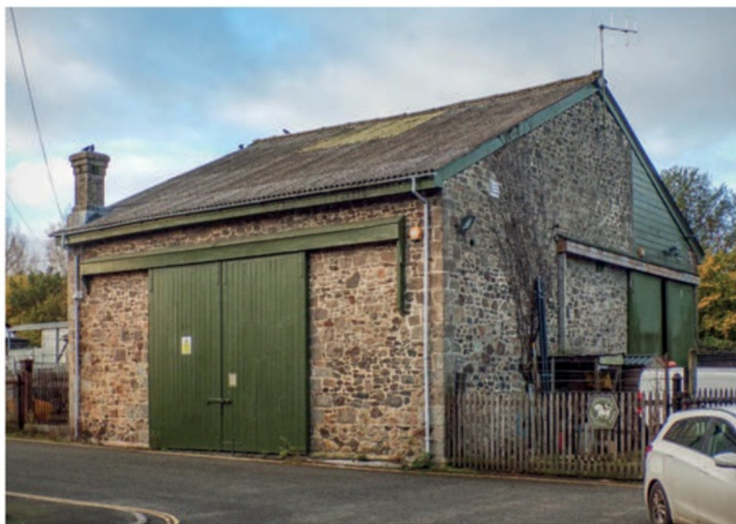
▲ A view of the still extant goods shed structure at Bovey, which currently serves as a store used by the Dartmoor National Park Authority. The station building also survives and now houses the Bovey Tracey Heritage Centre. The former trackbed through the station is now the route of the A382 town bypass. Visible just to the left of the goods shed is a GWR Toad brake van, which is one of a number of preserved railway artefacts displayed at the site. Photo: David Malton
