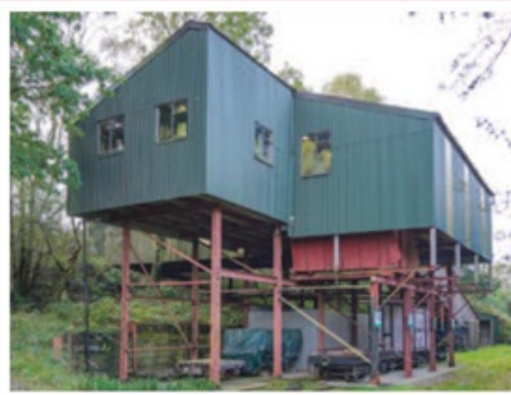
▲ The No.7 mine transshipment shed, which was donated by Imerys Minerals and re-erected at Norden, now forms the museum's main building.
