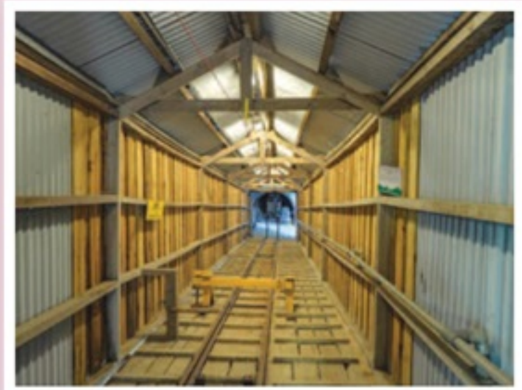
▲ Recreated at the site is this inclined tramway running from the mine adit, seen at the bottom. Clay was brought out of the mine in small tubs.
