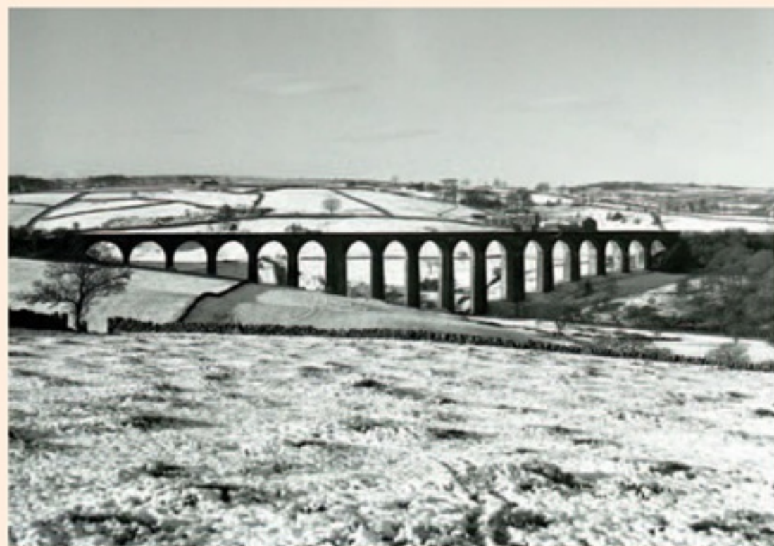
▲ A lovely study in the snow of Hewenden Viaduct near Cullingworth on the Keighley leg of the ex-GN routes which split at Queensbury. The viaduct survives today as part of the Great Northern Railway Trail, a right of way for cyclists, walkers and horse riders. Photo: R Wildsmith, Armstrong Railway Photographic Trust
