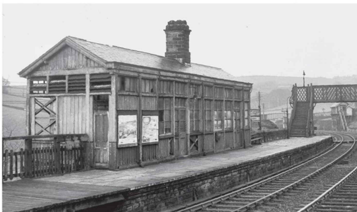
◀ The remains of the timber waiting room on the up platform of the Keighley-Bradford chord. Queensbury East Jct box is visible in the distance. Photo: The Transport Treasury
