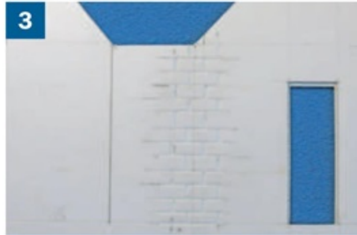
3 The stonework was scribed into the surface using a scraper board marker tool, which was held at an angle against a straight edge.
