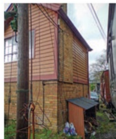
▶ A rarely-photographed view showing the rear elevation of the structure. Note how the brick fireplace protrudes slightly further than the locking room wall beneath it. Photo: David Malton
