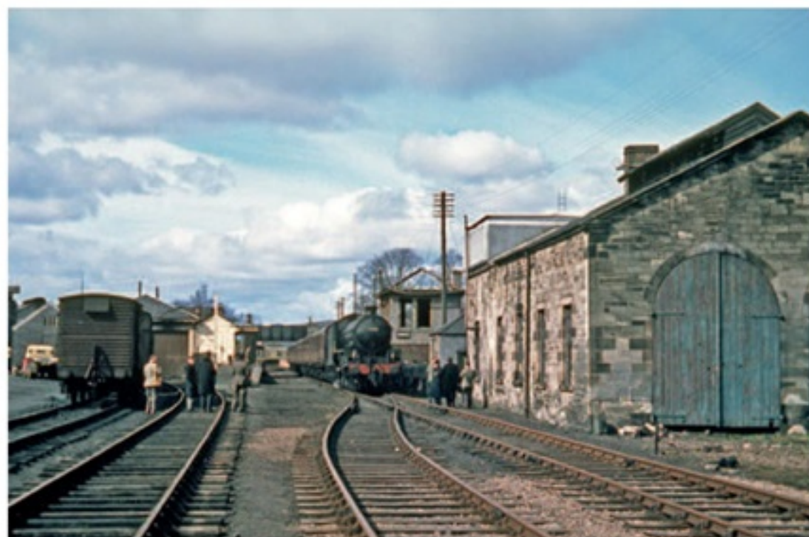
▲ Thompson B1 4-6-0 No.61324 is pictured at Duns on 14 April 1963 preparing to return to Reston with the Scottish Rambler No.2 railtour, which was organised jointly by the Stephenson Locomotive Society (Scottish Area) and the Branch Line Society. By the time of this photo the line between Reston and Duns was freight only: note the rationalised track layout and part-demolished signal box (visible to the right of the locomotive). Later that same day the railtour traversed the other remaining section of the Berwickshire Railway route between St Boswells and Greenlaw. Photo: Colour Rail
