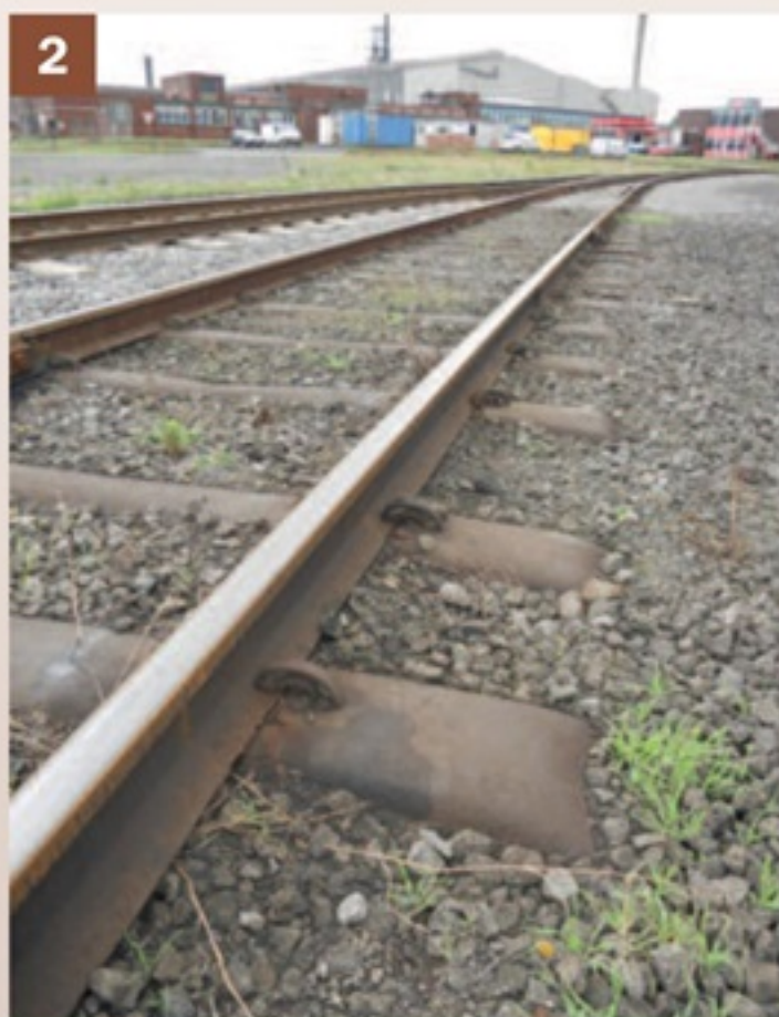
'Wisclips' were developed by the Workington Iron and Steel Company and were noted for their quick maintainence.
