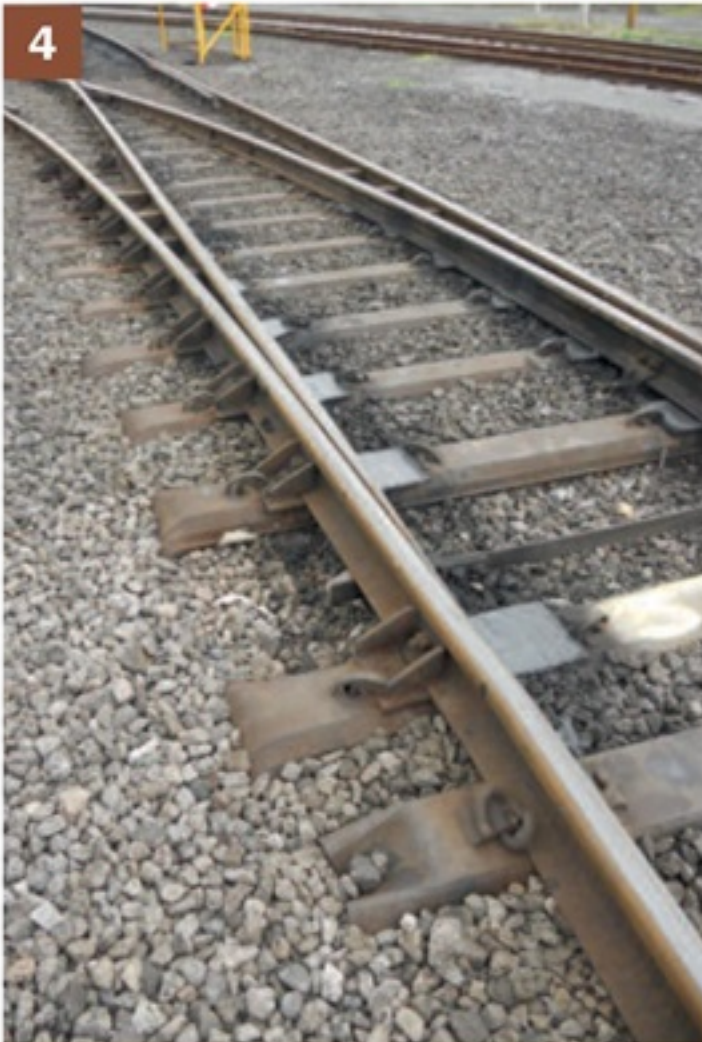
Points used fabricated steel chairs clipped to channels of varying lengths and a different cross-section.
