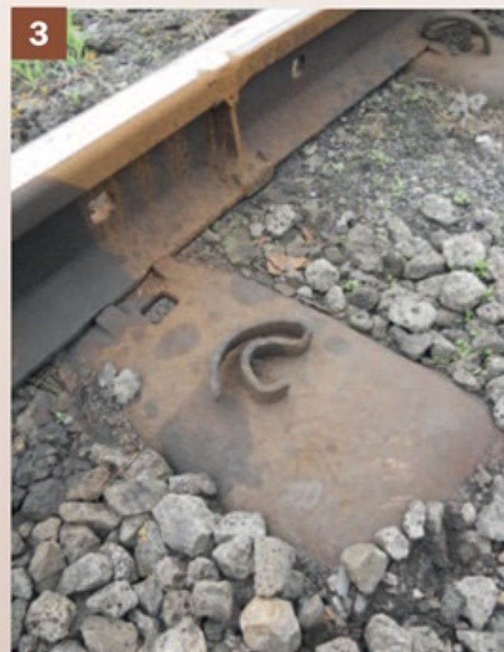
The Wisclip took the form of an exaggerated 'e' shape and was fitted into a rectangular hole in the channel.
