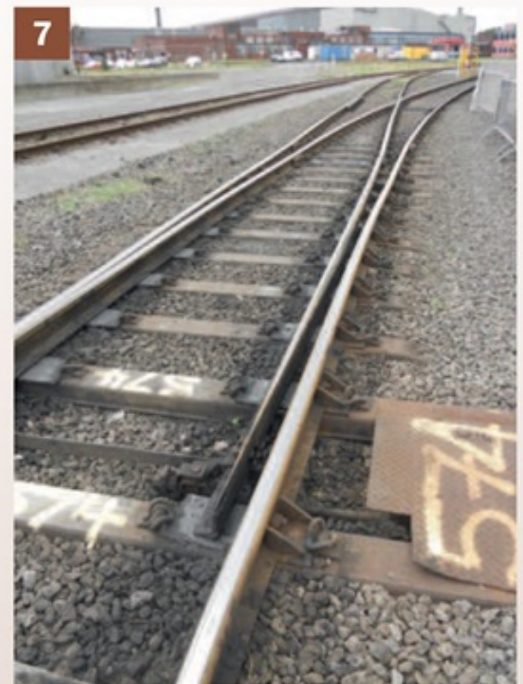
Channels were shaped to provide resistance to movement. The design is reflected with the Peco track.
