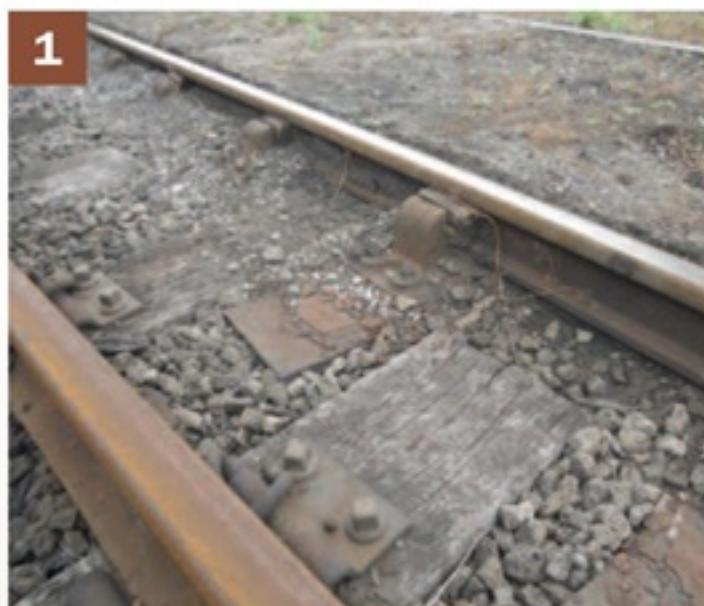
Early types of steel-sleepers often used modifications of fixings which were employed for existing track.
