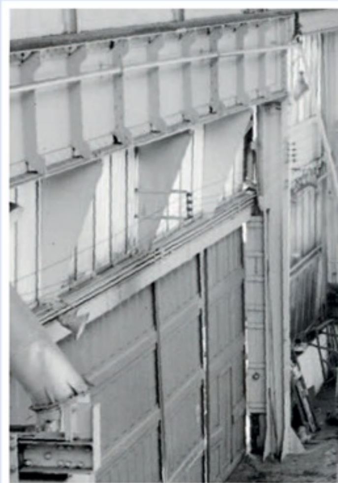
▲ The main erecting shop door which will be visible on the inside of the model. Also visible above it is the large crane track beam.
