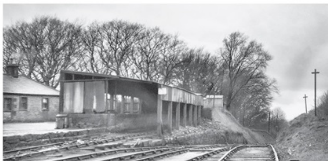
▲ The coal depot by the top of the incline provided fuel for the steam powered winding gear in the wheelhouse.
