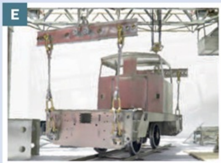
▲ The axleboxes are engaged with the horn guides and wheeling is complete.
