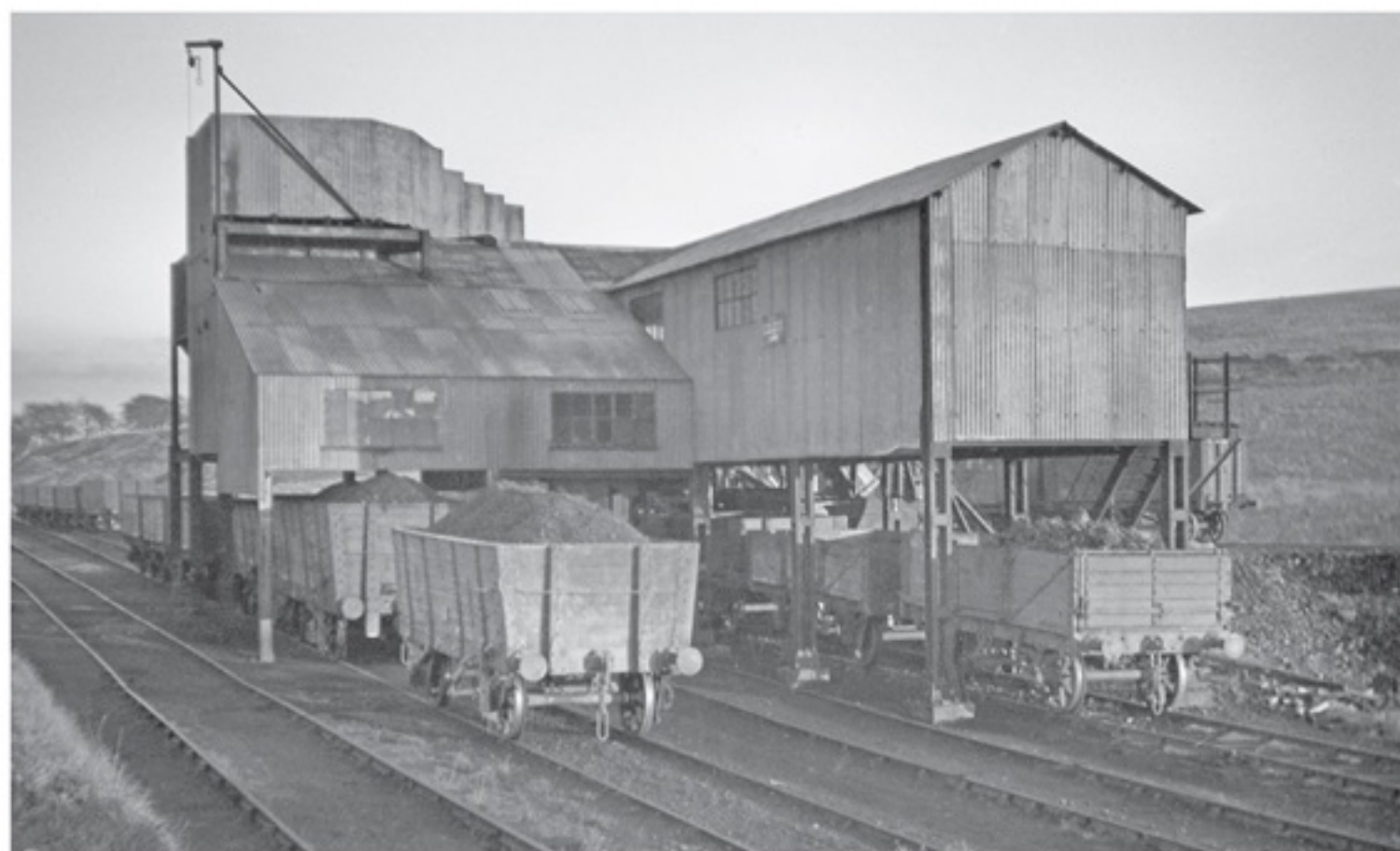
▲ Renewed hope of an increase in coal production in the 1930s resulted in the construction of this loading structure. Known as the Howard Screens they were built on the site of some earlier workings about 800yds to the east of Hallbankgate. Seen here in NCB days in the early 1950s, they appear to have been in use up to the time of the railway's closure, although they were demolished soon after. They are not shown on the proposed layout plan, though could easily be added at the lower right in place of the traverser if space permitted.
