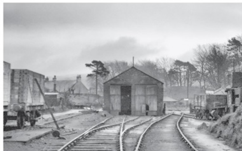
▲ The two road loco shed looking slightly worse for wear. Beyond are the two road crossings, where the 'whistle' signs are located. Some gate posts can just be seen, though evidence as to if and when any gates were ever fitted, is not readily available.
