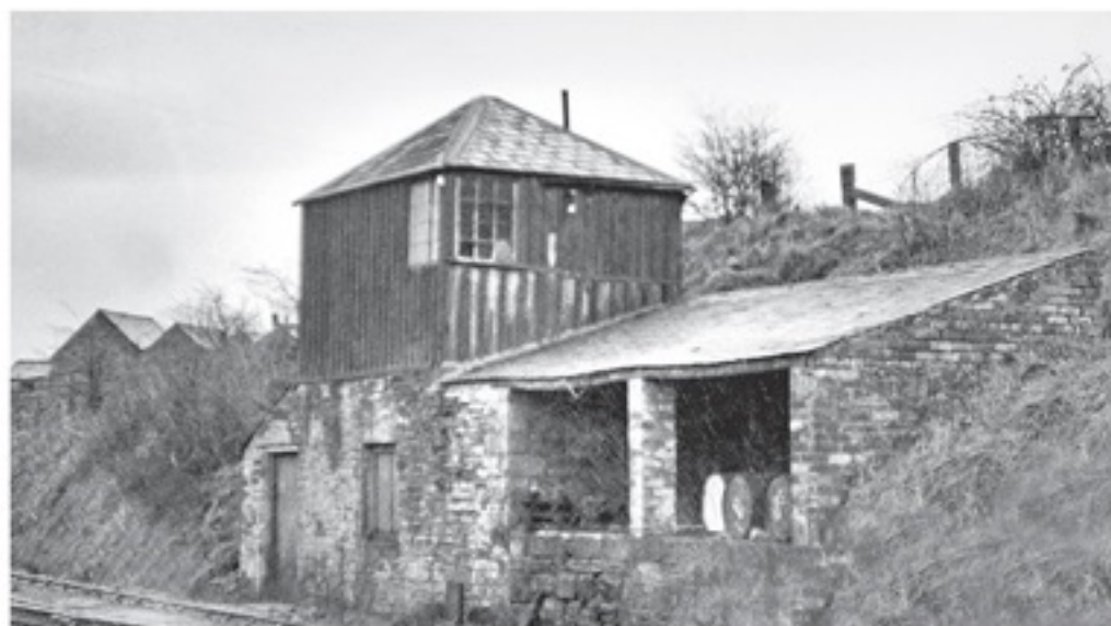
▲ The incline wheelhouse or 'control room' is reputedly to be a design of Robert Stephenson's from the early 1830s. It was possibly out of use at the time of closure in 1953, as other photographic evidence suggests that 20th century steam power could handle the gradient with short trains.
