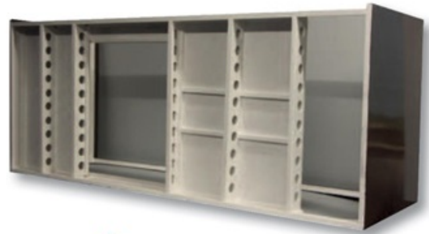
▲ A view of the 'box' from the underside showing the timber and plywood construction.
