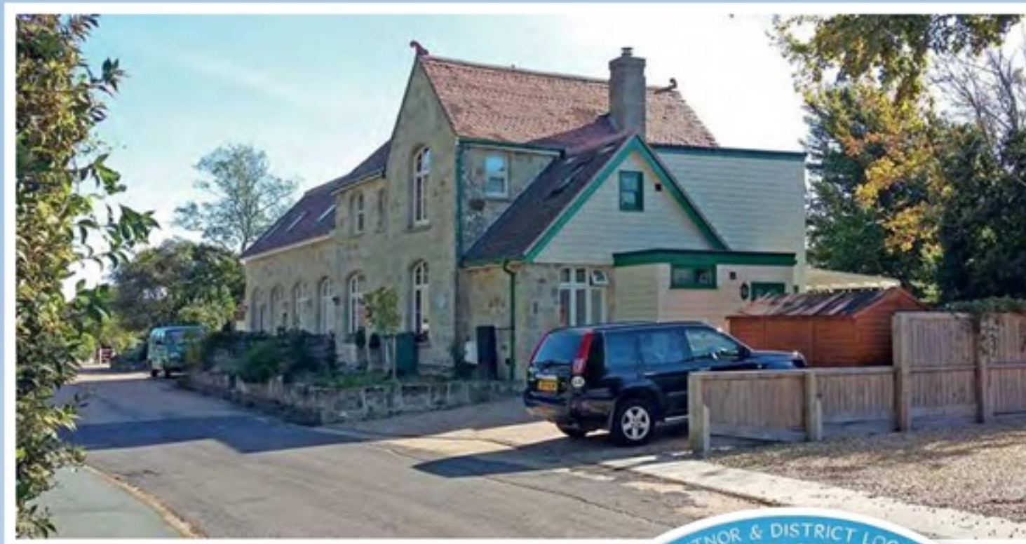
▲ A view from what was the platform side of the former station building, with the plaque affixed to it pictured (inset). Photos: author
