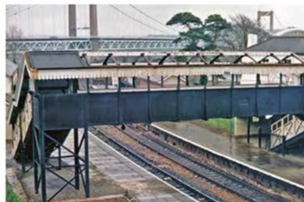
▲ The footbridge seen from the up platform. The suspension road bridge and the tubes of the Royal Albert Bridge are in the distance.
