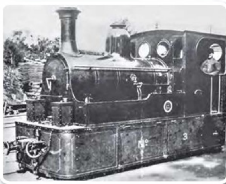
▲ Castlederg & Victoria Bridge Tramway No.3 was built in 1891 by Kitson & Co. The tramway skirts avoid the need for an accurately modelled running gear. Photograph: author's collection
