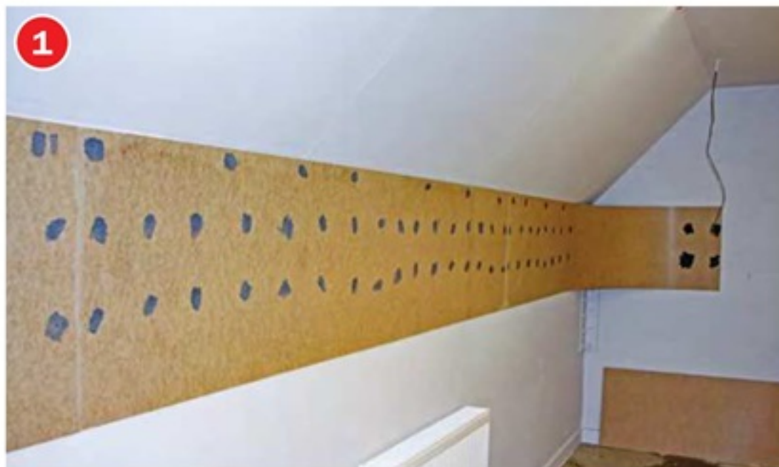
▲ The first task was to install the backboard for the backscene. This was simply hardboard nailed to the plywood wall with grip nails. The hardboard was curved around the corners.
