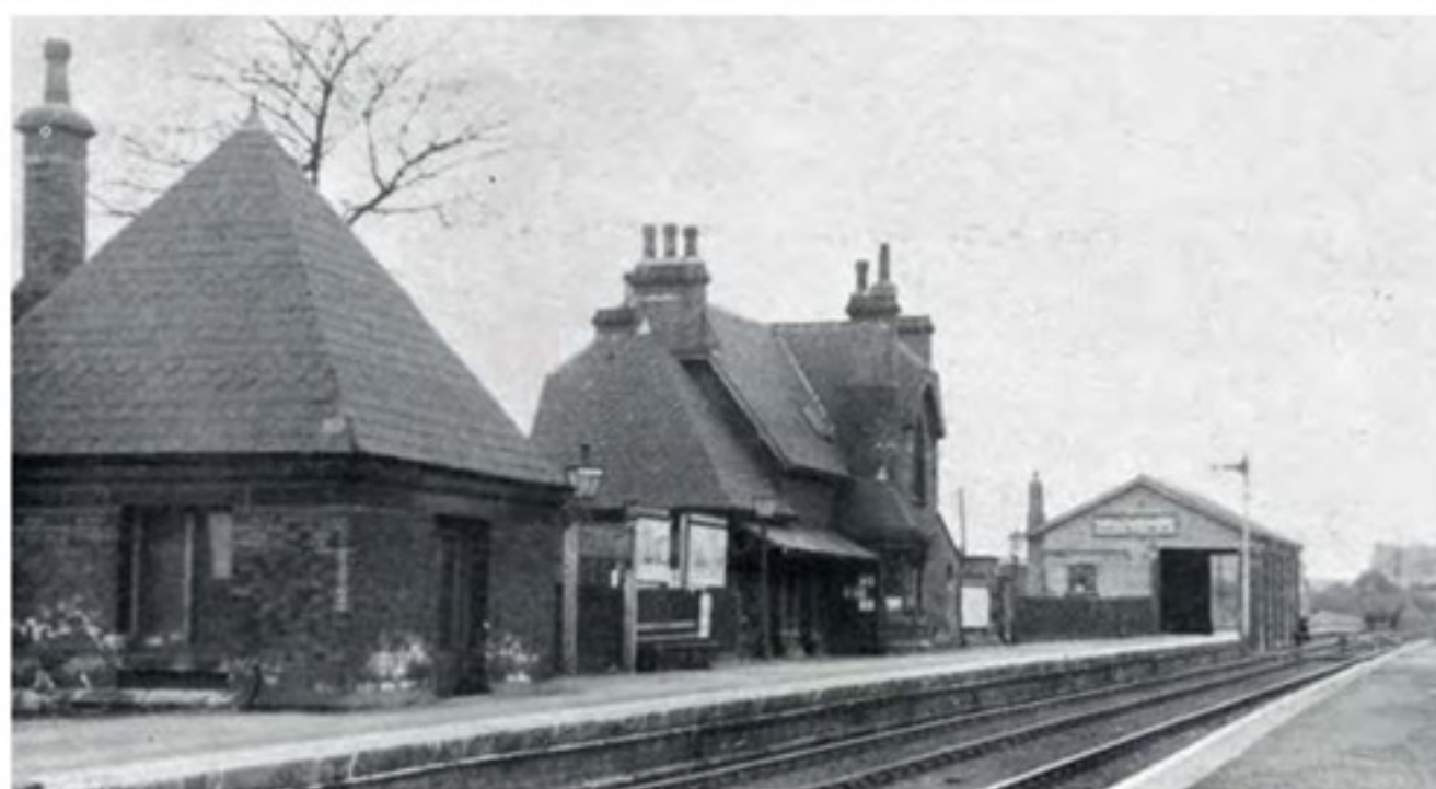
▲ The goods shed was a conventionally-designed structure, unlike the station building and porters' room; it is visible in the background of this undated photograph.
