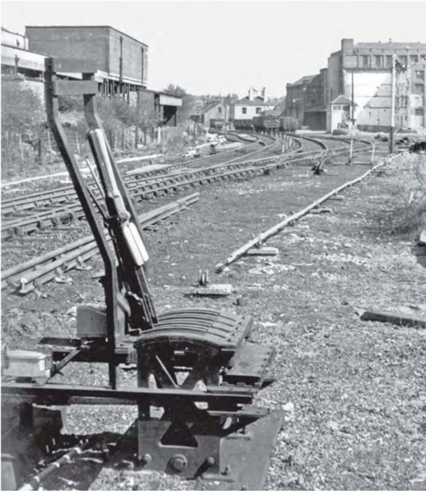
▲ A general view taken just before the MS&L signal cabin was closed, to be replaced by the ground frame in the foreground. Several empty and loaded 16T coal wagons can be seen in the Co-op sidings and beyond the dominant Co-op warehouse. Photograph: author's collection
