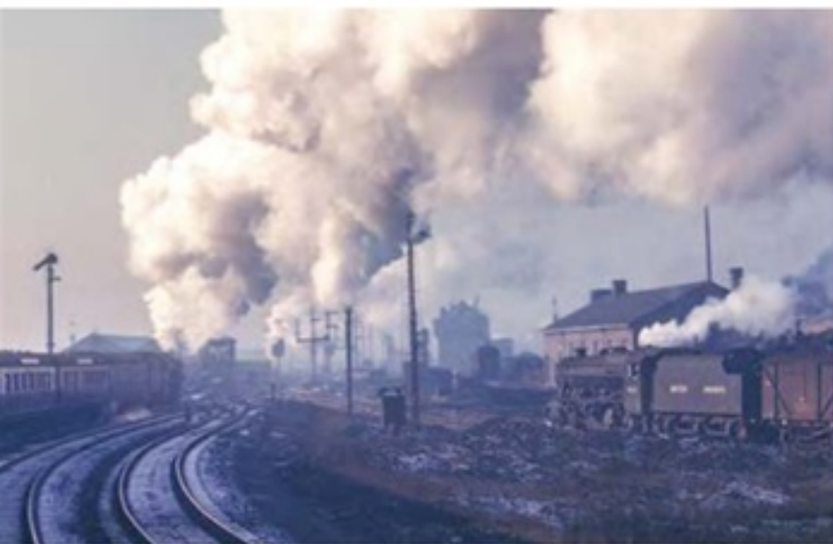
The real thing – a frosty January 1949 morning sees lots of steam plumes as a Princess Coronation class loco departs Crewe on a Bristol bound service and not a diesel in sight. Photo: Frank M Owner
