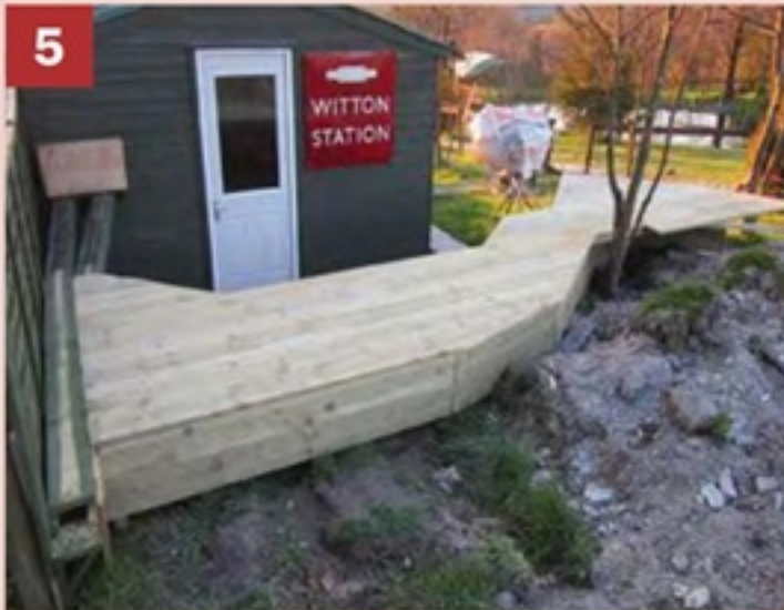
▲ The decking is almost complete, April 2013. The hatch to the left of the door...
