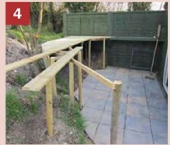
▲ Supports and planking were assembled from treated timber.
