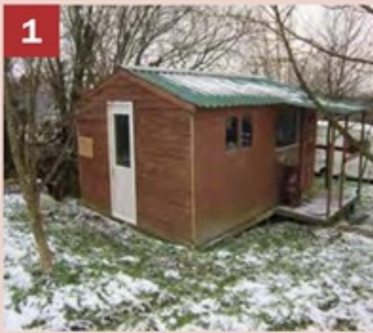
▲ Construction began during winter 2012/3. The bank (left)...
