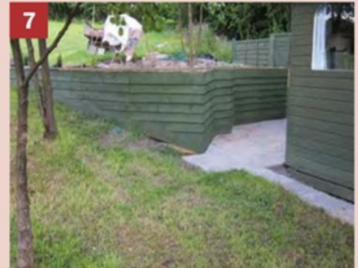
▲ By July 2013, panelling had been installed to tidy the appearance, and painted.
