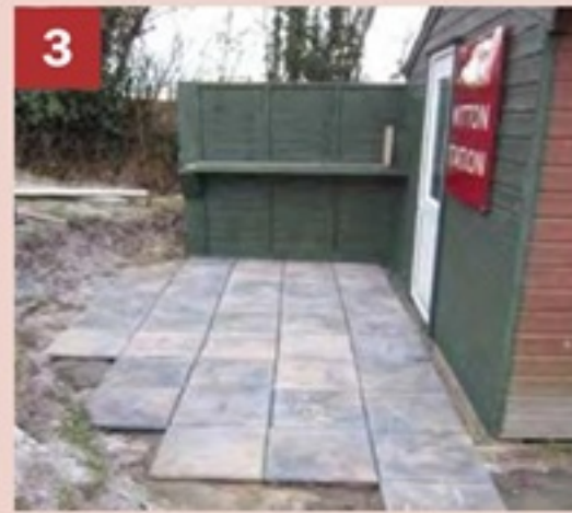
▲ Once the site was level, paving slabs were laid. April 2013.
