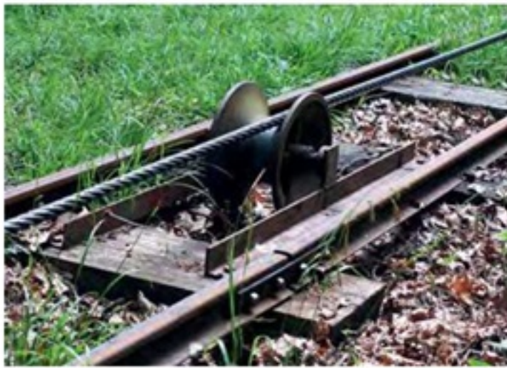
▲ The cable runs on rollers set between the running rails, interspersed with pulleys to keep the cable centred.
