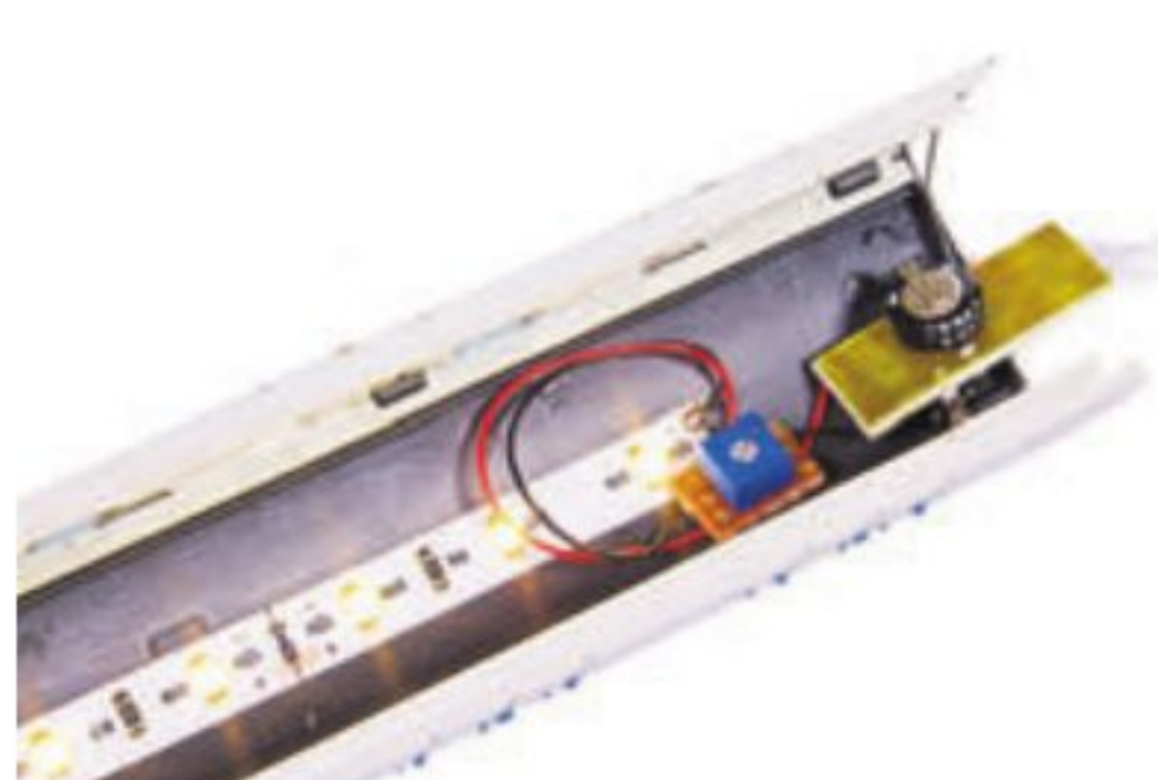
Two wires connect the circuit board to the lighting strip - black to the negative terminal and red to the positive terminal. The kit is tested before installation by removing the backing paper from the lighting strip and securing with the self-adhesive backing.
