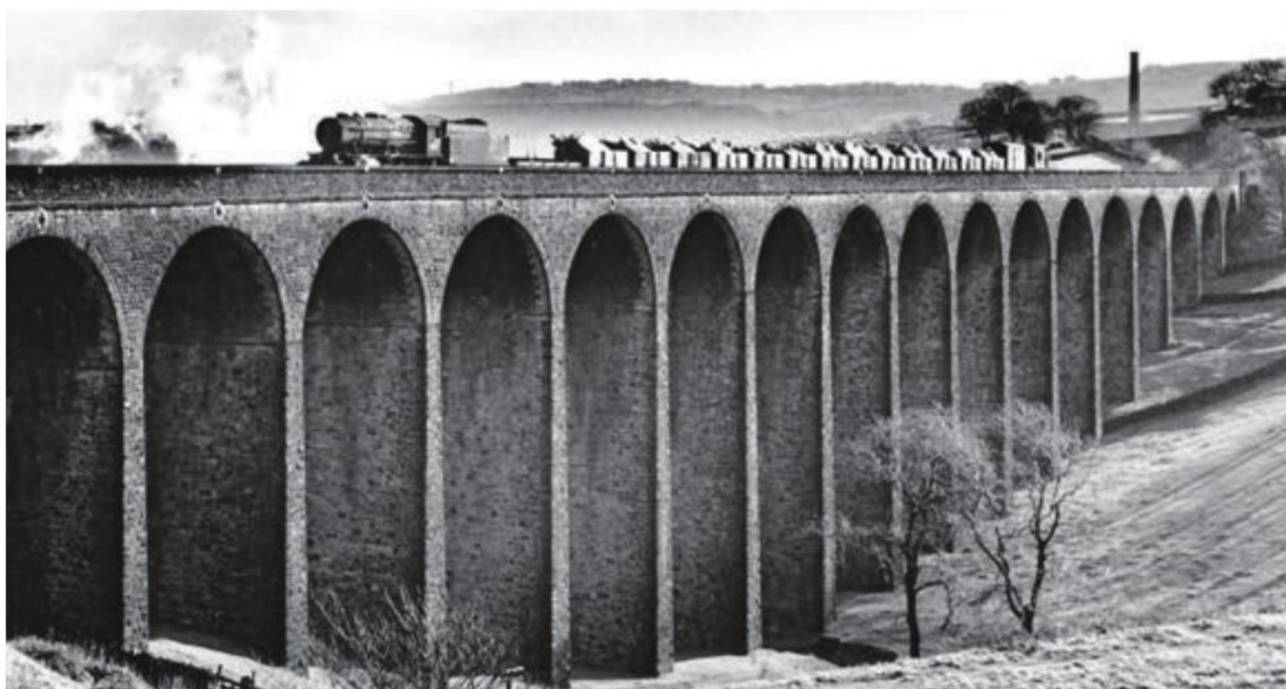
Thornton viaduct, one of three viaducts on the Queensbury Lines.
