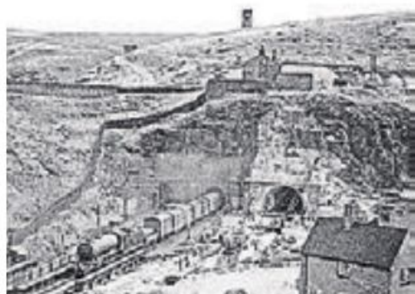
Photograph from 1953 showing the western portals of the Woodhead tunnels. To the left, a train emerges from one of the original tunnels, while tunnel three is under construction to the right.
