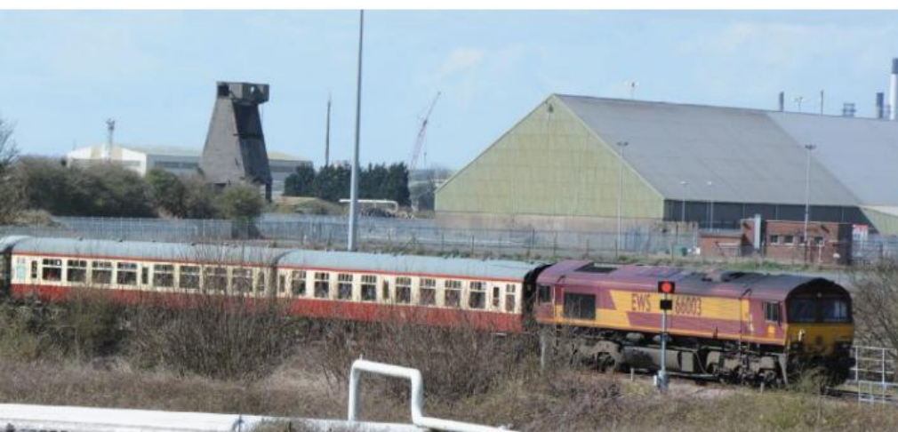
The coal tower still stands at Immingham as can be seen in this modern-day shot. BRIAN SHARPE
