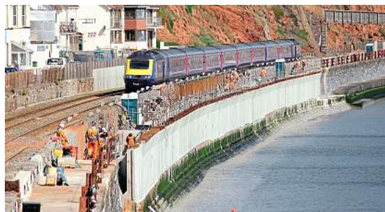
REPAIRS to the Dawlish sea wall – which was damaged in February 2014 – are nearing a conclusion. On March 24, HST No. 43024 leads a set passing Riviera Terrace with the 9.06 Paddington-Plymouth service. STEWART ARMSTRONG
