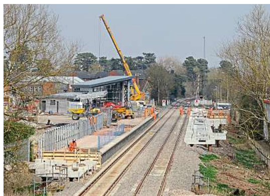
BICESTER VILLAGE: Construction of Bicester Village station is beginning to take shape. This view on April 10 shows a much more substantial affair than previously envisaged. CHRIS BEHAN
