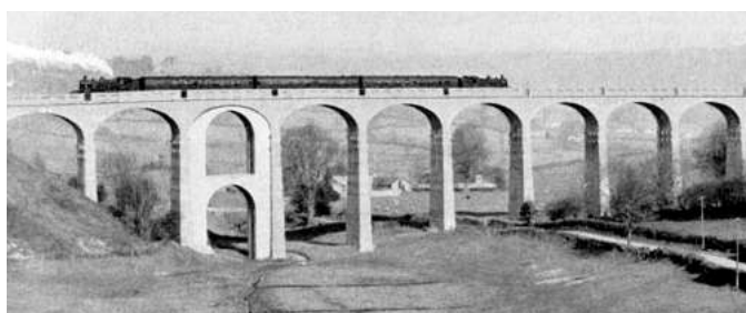
The Lyme Regis section of the 'East Devon Rail Tour', topped-and-tailed by 41291 and 41206, crosses Carrington viaduct in 1965. See feature starting on page 20.
