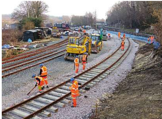
Looking towards the RVR and NR's respective stations on March 20, the new main line connection is via the track in the immediate foreground. PETER BROWN
