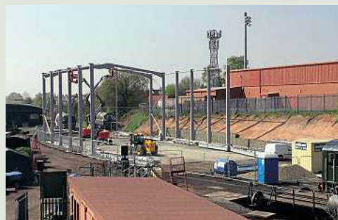
CONSTRUCTION of the Severn Valley Railway's diesel depot and lifting shop was well under way in April. The 1,000 sq metre, two-road structure is being built at the station end of Kidderminster carriage shed (visible on the left). BOB SWEET
