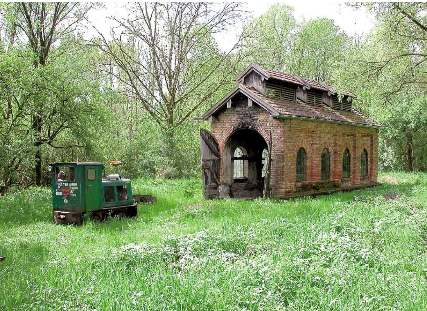
Like a scene from a fairy story... the engine shed of the Füglein Peat Works Railway, still in daily commercial use despite its almost mythical appearance.
