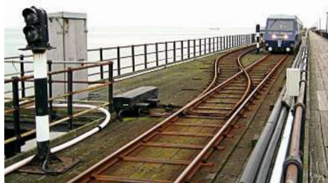
Southend pier features a conventional signalling system, this one controlling a passing loop. NICK PIGOTT
