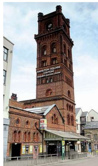
The exterior of Hamilton Square station on Merseyside. NETWORK RAIL
