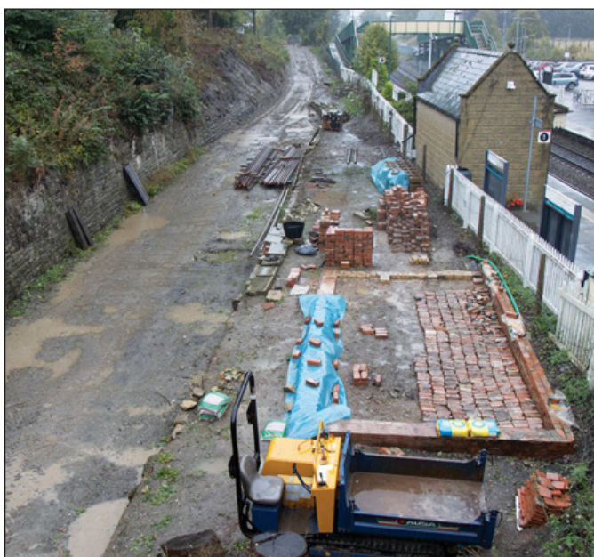
■ Much progress continues to be made on the revival of the Glyn Valley Tramway, the Chirk station site now completely clear, the footings of the station building being worked on and clearance spreading along the trackbed. Tracklaying is expected to start soon and NGW hears this is now intended to be laid permanently to 2ft 3in gauge. We hope to bring more details soon, our planned feature for this issue on the revival project having been delayed by bad weather. Photo: Andrew Charman
