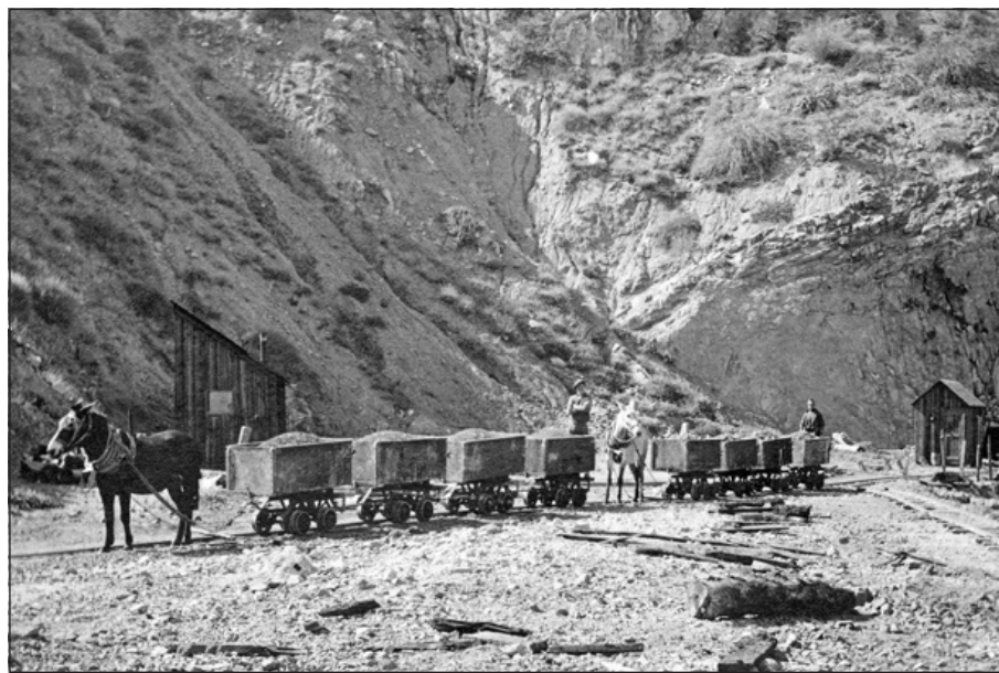
Above: The 2ft gauge tramway on Level 10 of Engels Copper Mine which ran to the top of the Superior mill. One of the 7-ton locos is hauling a train of heavy ore cars. The line crossed more than 1,100ft of trestles. Photo: Dan Quine collection
