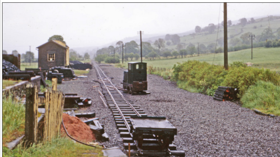
Above: Looking the other way from the previous picture – points are installed for future sidings and the line stretches towards Bala.
