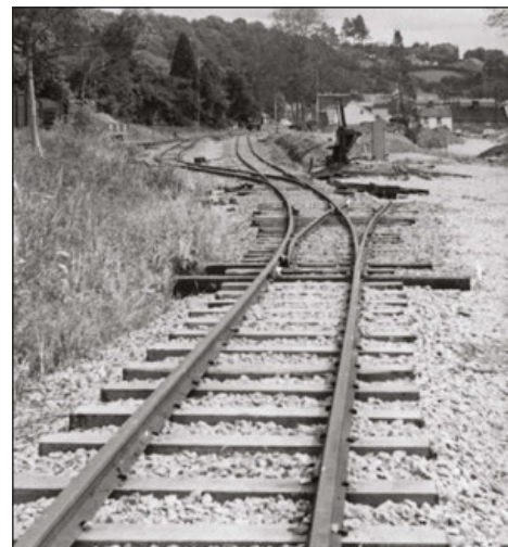
By early 1981 a brand-new station was steadily emerging from a field at Raven Square in Welshpool.
