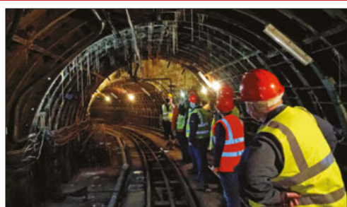
■ MAIL RAIL TUNNELS – ON FOOT
