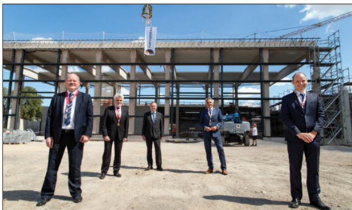
A host of guests witnessed the topping out of the new building, including Saxony transport minister Thomas Webel who signed off the project in the Autumn of last year. Photo: HSB
