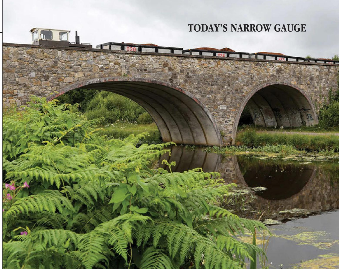
Above: The attractive Rathdrum viaduct over the Grand Canal on the Derrygreenagh system. A loaded rake is on its way to the Croghan tippler in August 2016.
