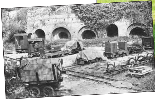
Right: The embankment for the demonstration line built by volunteer navvies with much sweat and effort was never finished before the move to Amberley and now appears to be part of a motorbike scrambles circuit.
