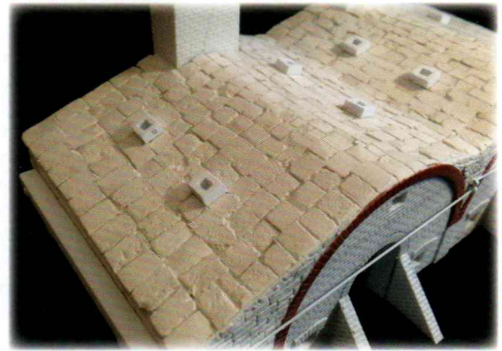
Right: Close up of the roof tiles. These were fired clay tiles set in mortar with a series of roof vents. These could be closed off with a small tile and were used to control heat. Powdered coal could also be dropped into these to aid the firing process.
