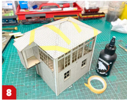
8 The roof panels were then bonded to the trusses, again using PVA to allow time for adjustment. I later cut the porch roof extension away to make it easier to add the roof slates...
