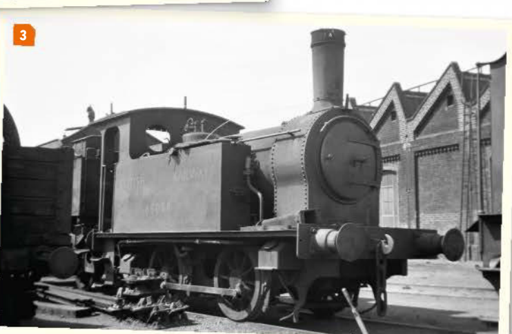
3: No. 68088 also boasted spark arresting apparatus atop the chimney, a legacy from its time working at Tyne Dock. It is seen at Stratford in August 1949 and it looks like the enclosed rear cab sheet has been partially removed. D. WILLIAMS ARCHIVE/RAIL ONLINE
