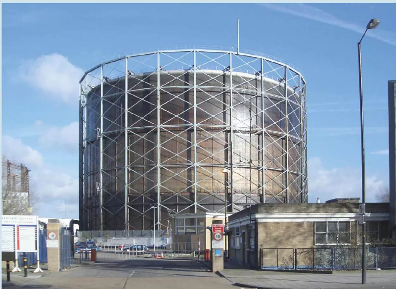
Above: The 'Number 13' holder, seen here in 2006 while it was still operational, at the Old Kent Road Gas Works site. As you can see, it's a substantial structure and, when it was built in 1879-81 it was the largest in the world, although many erected since then were even larger. It was 160ft tall with a diameter of over 210ft and could hold 5.5 million cubic feet of gas and featured 22 wrought iron standards (columns). Although it is still standing, being Grade II-listed, it is now decommissioned. PHIL SUTTERS
