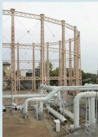
Right: This is a smaller lattice frame-guided gas holder at Battersea. Note the crown of the holder is at ground level and there's a jumble of large-scale pipes in the foreground. Next to it was the infamous rigid type gas holder 'Number 7' that was an iconic landmark and dominated the skyline over Stewarts Lane Depot. Built in 1930-2, this structure stood 295ft tall and could hold 6.5 million cubic feet of gas. All the holders on this site succumbed to demolition at the end of 2017. GRAHAME HEDGES
