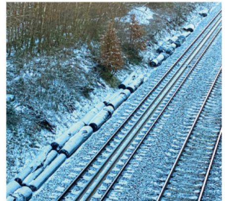
Below: Near the western portal of Cowburn tunnel, on a bitterly cold afternoon, rolls of what appears to be waterproofing material have been stockpiled in the cess, while long lengths of new rail have been dropped ready for renewal work. GEORGE DENT
