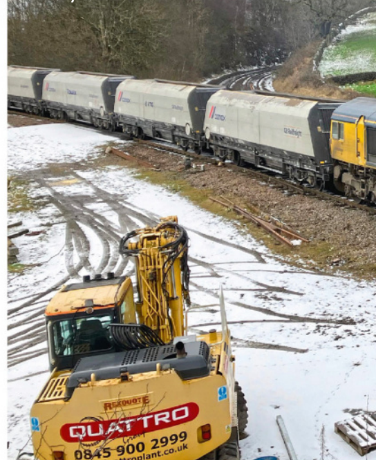
A very dusty 66701 restarts the 6E51 Peak Forest-Selby limestone hoppers at Chinley East Junction on January 16. GEORGE DENT
