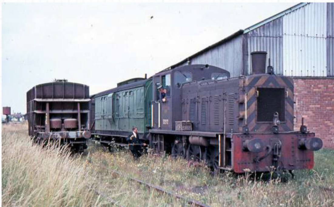
Above: The Food Buffer Depot, built in the early 1950s at Wheldrake, handled stores of sugar, corned beef, flour and biscuits, stockpiled in case of national emergency or nuclear war. Further back towards the station was a row of eight post-war Nissen hut warehouses, although only four have been included on my model plan. This colour image was captured in July 1964. GEOFF LUMB/DAVID MITCHELL
