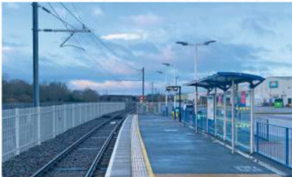
Above: Rotherham Parkgate Station, looking towards Rotherham Central. Note the mast on the opposite side so as not to encumber the platform, and also note that it’s placed outside the boundary fence.
