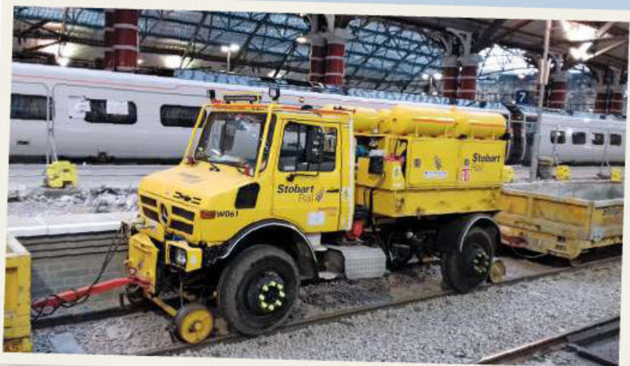
A Stobart Rail Mercedes-Benz road-rail Unimog, coupled to a pair of trailers, is seen at Liverpool Lime Street during platform upgrade works in February 2018. GEORGE DENT
