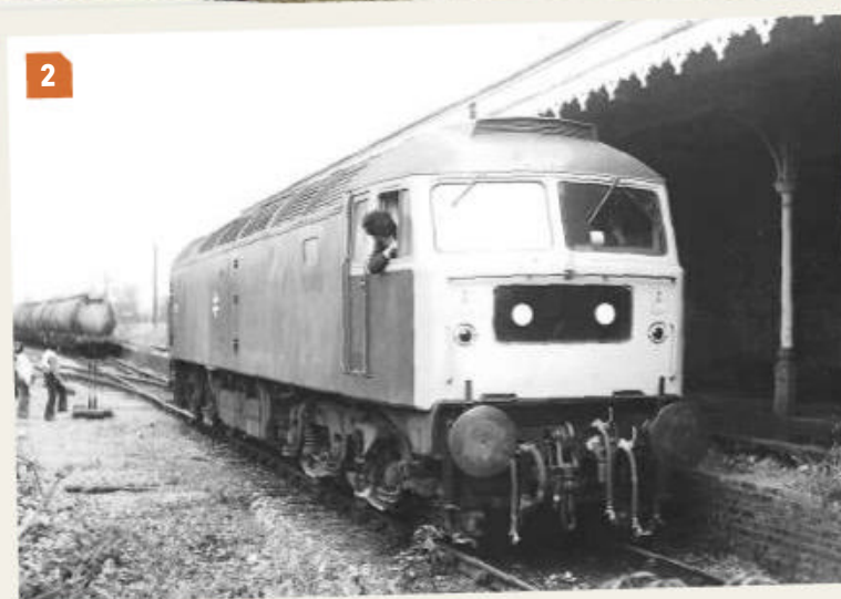
1: The Serck shutters have opened as 47223 recovers from a signal slack at Iwer with the Langley-Lindsey refinery aviation fuel empties c.1991. It has standard marker lights at this end. CHRIS LEIGH
