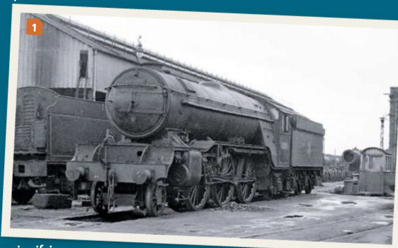
1: Paired with a GWR tender in the equally unlikely surroundings of Swindon Works, 'V2' No. 60845 was undergoing coal consumption trials on the Western Region in March 1953. RAIL PHOTOPRINTS
