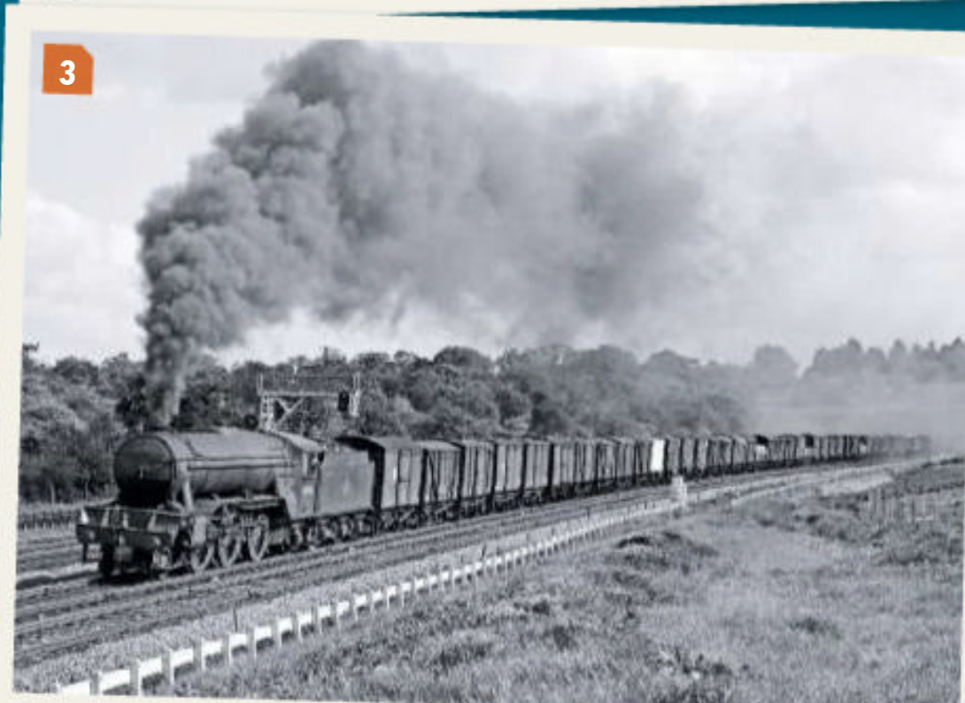
3: The ungainly addition of outside steam pipes reveals that No. 60956 has lost its monobloc cylinder casting. The scene is captured at Hadley Wood North in 1959. RAIL PHOTOPRINTS
