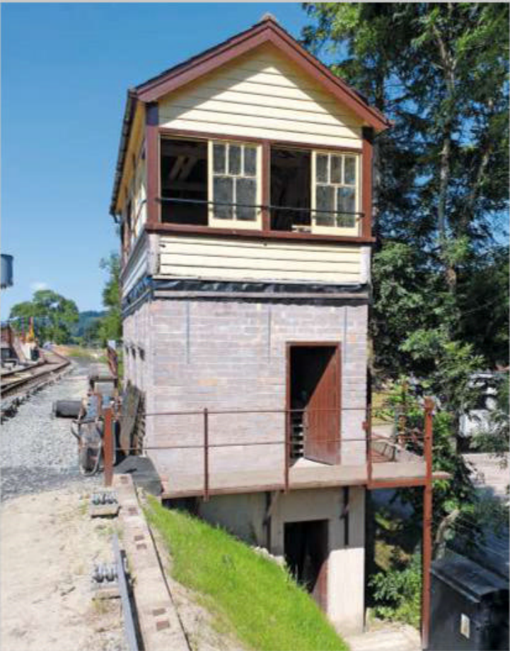
Above and right: The upper section of the signal box is from Weston Rhyn; it's been a complex build on three floors.
