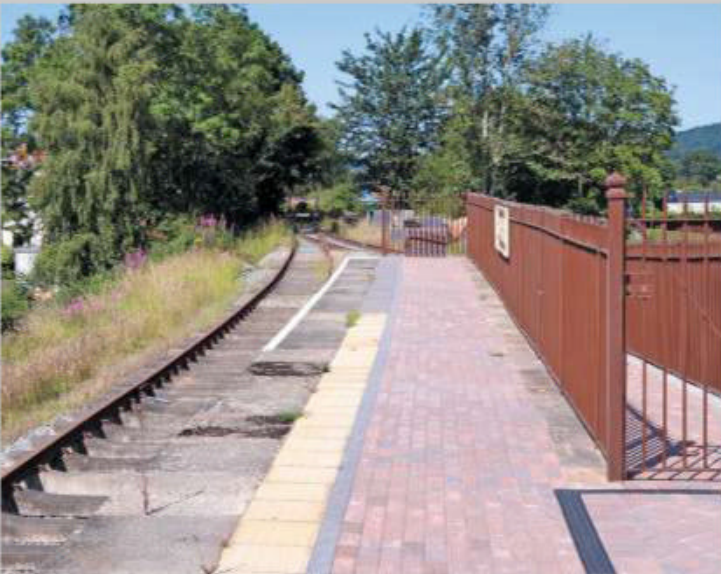
Below: Where possible, Llangollen has used recycled materials. The platform edging slabs on this side came from Bala Junction Station; those on the other face came courtesy of Network Rail.
